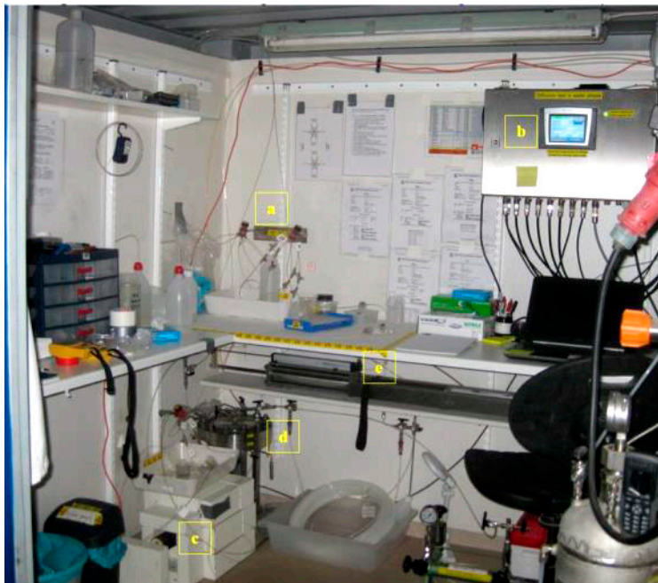
Figure 2-3. Container in the REPRO niche, containing equipment such as sampling- and injection loops (a), data taker (b), online detector (c), pressure regulation unit (membrane chamber; d), and piston pump (e).
