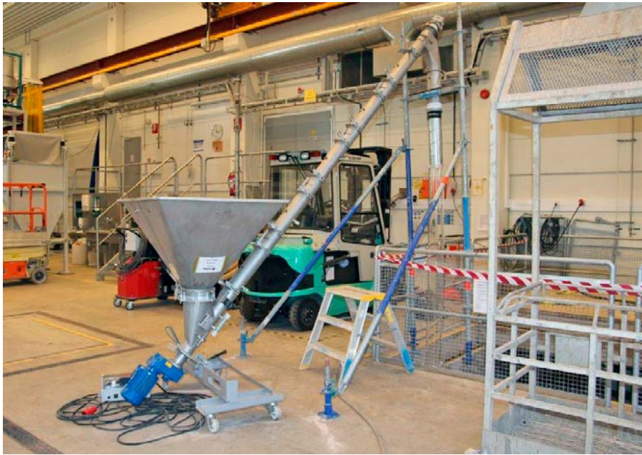
Figure 7-4. Photo of the conveyor screw with a hopper. The simulated borehole ends up two meter above the floor level.
