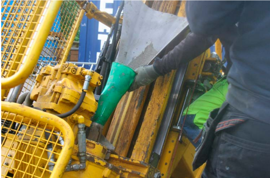
Figure 12-7. The concrete was manually poured into the drill tubes.
