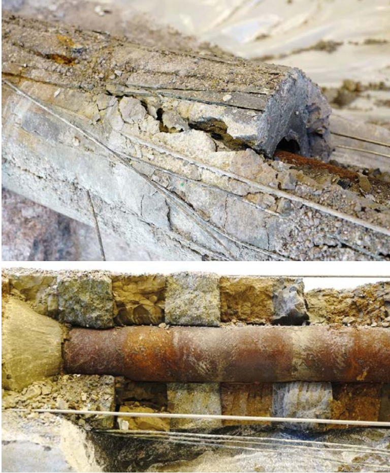
Figure 3-27. Highly fractured bentonite blocks from the very high temperature experiment ABM5 excavated in 2017.
