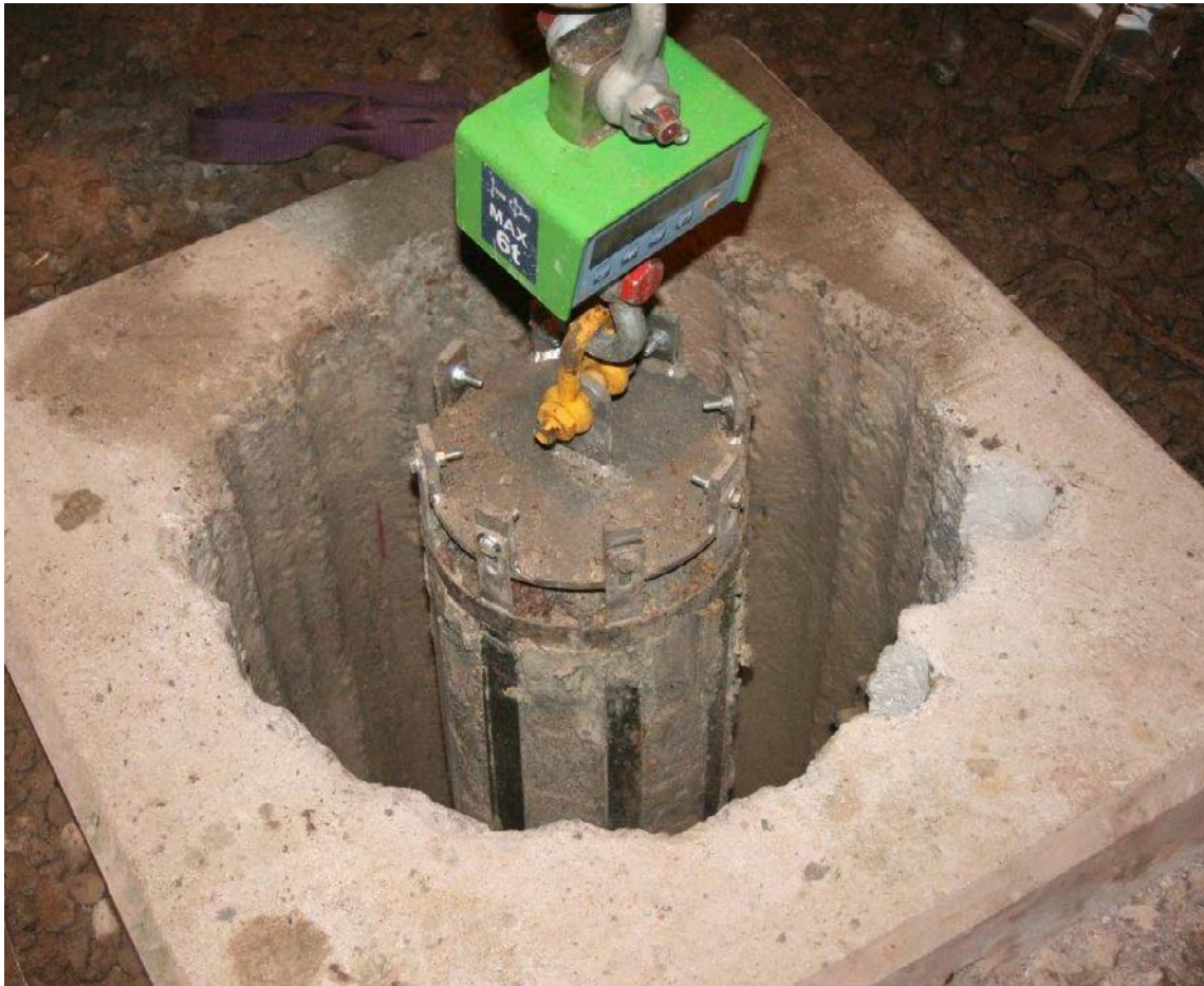
Figure 3-25. Lifting of the bentonite package.
