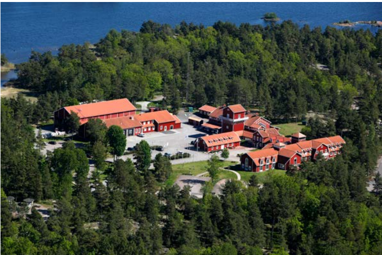
Figure 6-6. Äspö HRL above ground office buildings.
