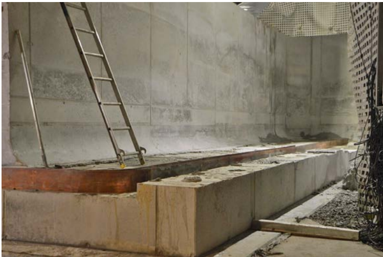
Figure 3-15. Section 1 just after demoulding.
