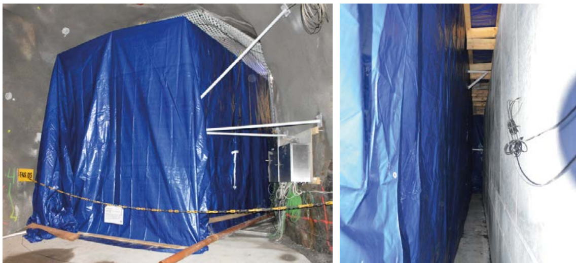
Figure 3-17. The tent-like structure covering the concrete structure during the stress test.
