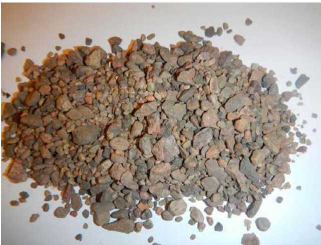
Figure 10-7. Photo showing the gravel used in the gap between block and rock.
