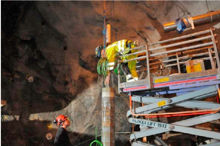
Figure 10-3. The blocks were threaded onto the steel tube one by one.
