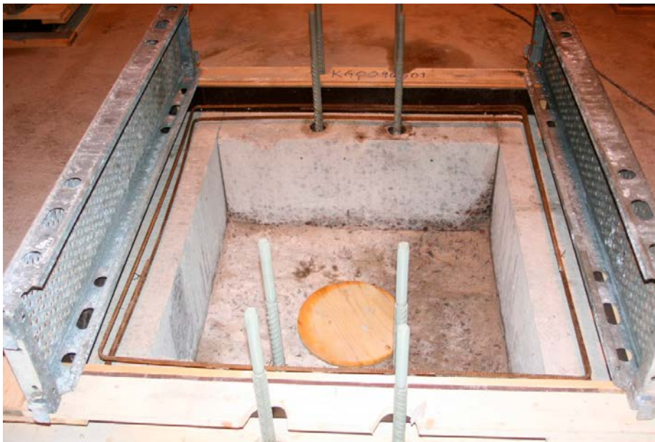
Figure 10-1. Preparatory work at test site.
