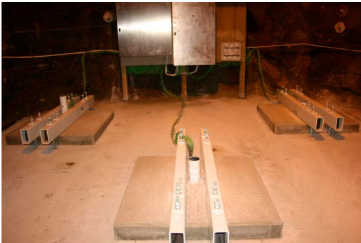
Figure 10-9. Photo showing the three test packages after finishing the installation work.
