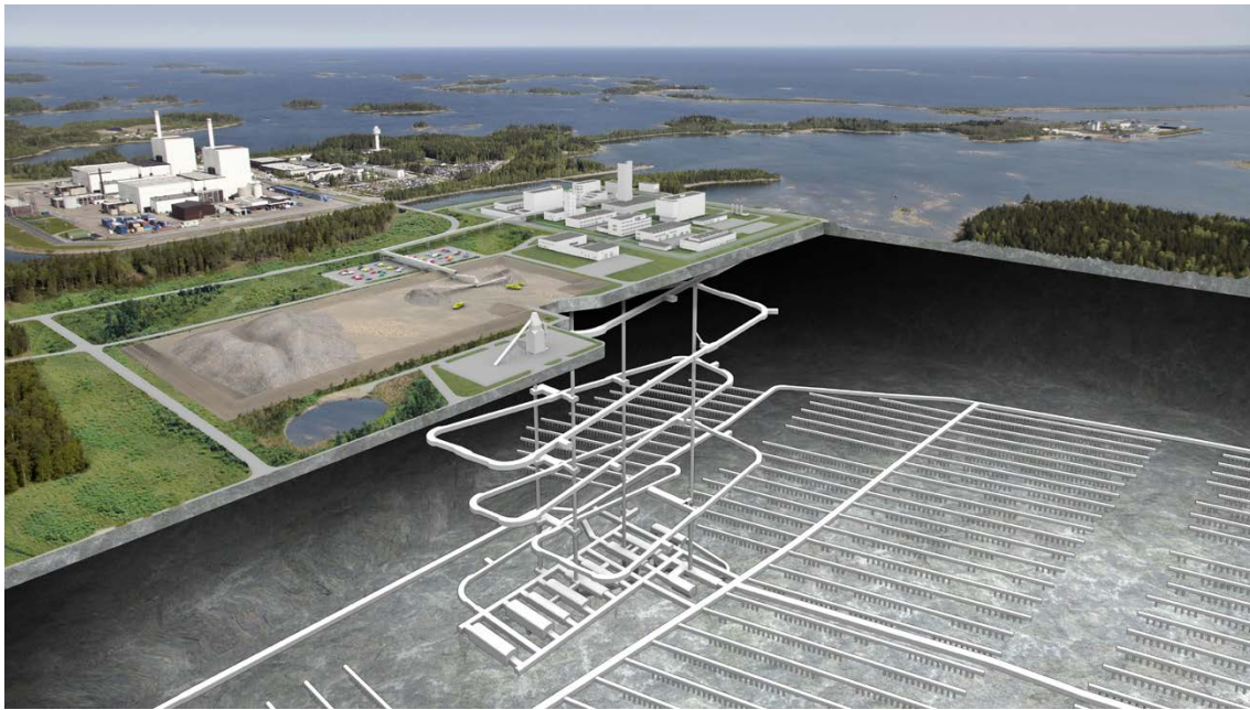
Figure 2-2. Parts of the final repository viewed from the north, showing accesses (four shafts and a ramp) between facilities above ground and the central area at repository depth.
