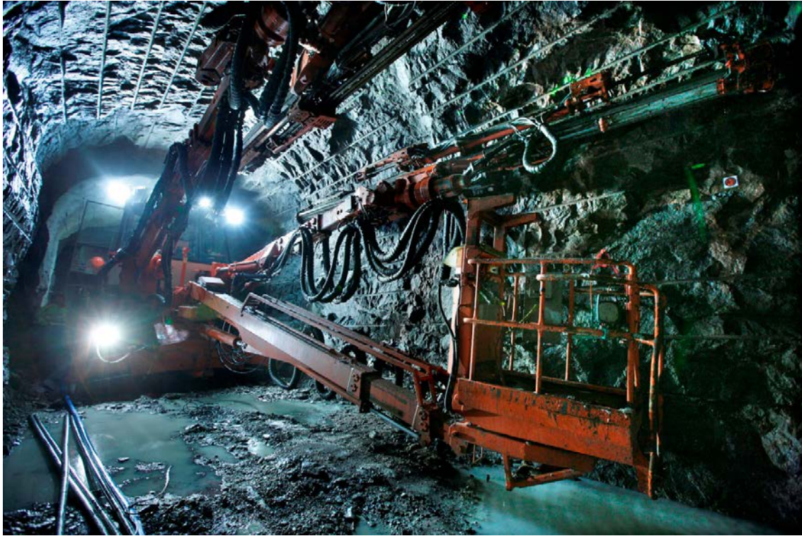
Figur 5-3. Borriggen (Sandvik DT1121i) under arbete i tunnel TASN.
