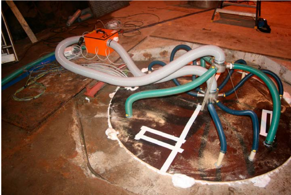
Figure 4-1. The top part of the deposition hole used for the test.
