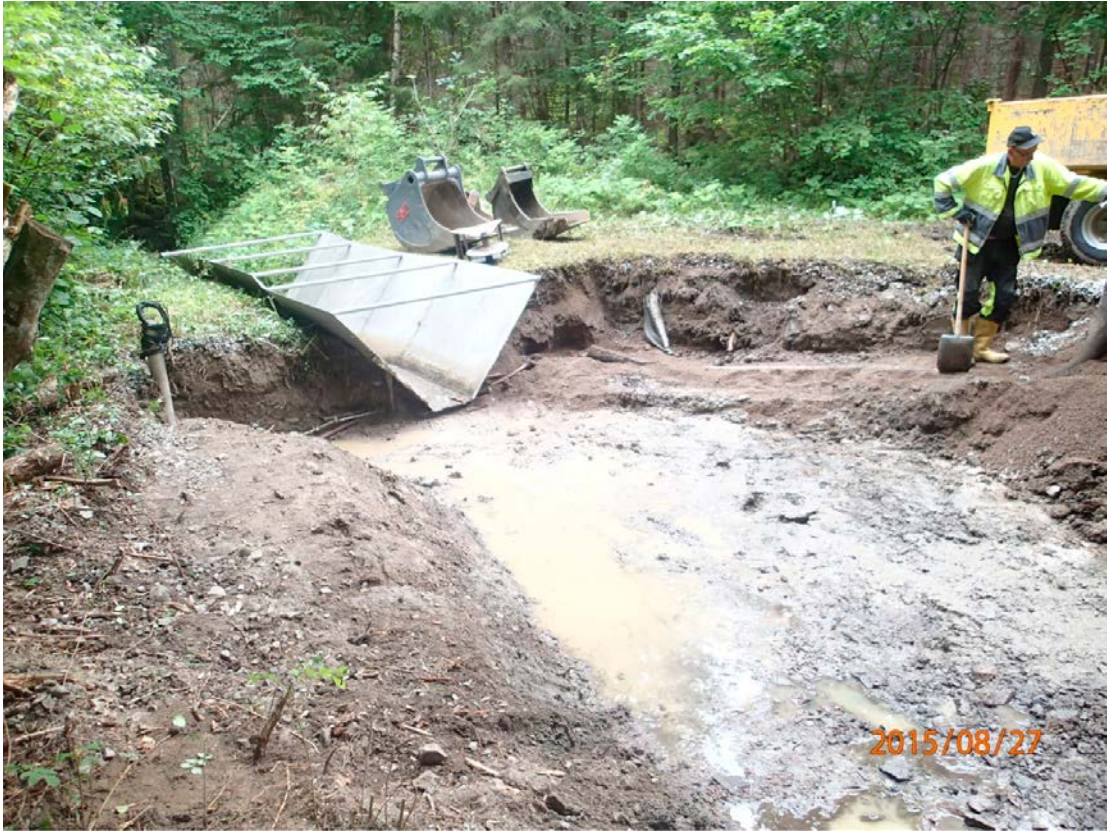
Figure 2-1. Excavation of the pool between the two flumes at PFM002669.
