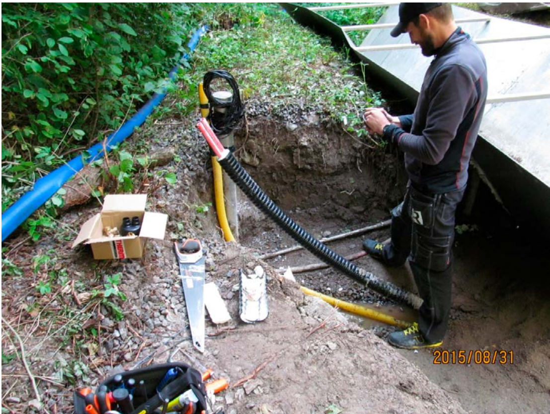
Figure 2-2. Installation of the heater system at PFM002669.
