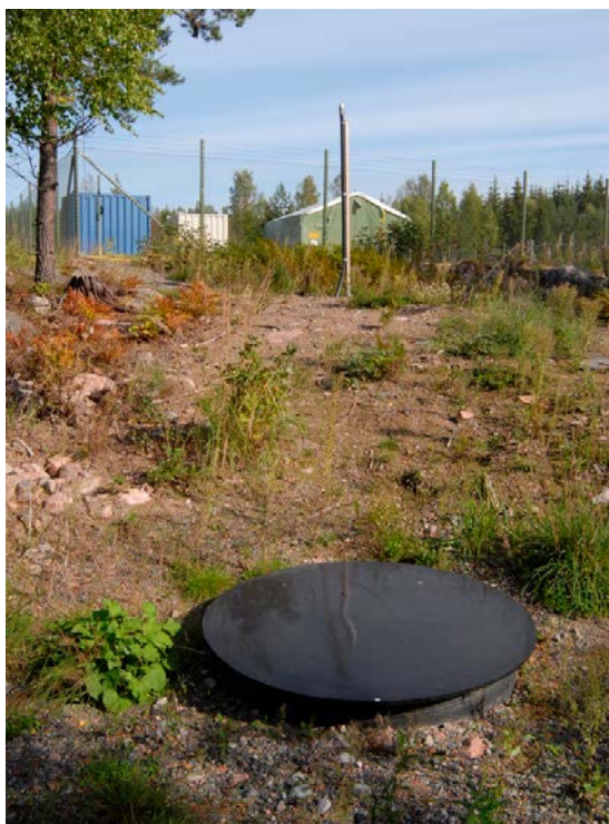
Figure 4-2. Top of concrete silo containing the SNSN seismic station near drill site 4 at Forsmark.
