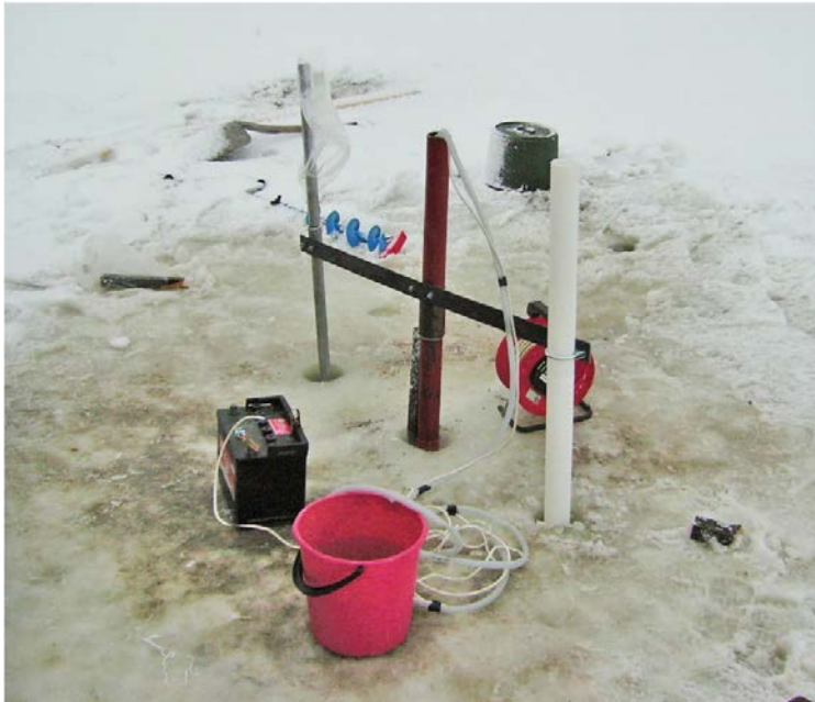
Figure 6-18. Groundwater monitoring well SFM0081 (middle), BAT filter tip SFM0082 for pore pressure measurements (left) and BAT filter tip SFM0083 for water sampling (right), installed below open water in Lake Bolundsfjärden. The picture shows sampling from the ice during winter.
