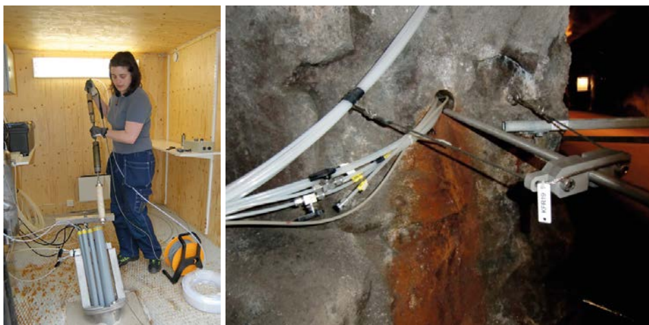
Figure 6-30. The core-drilled boreholes drilled from the ground surface are sampled (left) by pumping in the stand pipe. The equipment which is lowered in the standpipe consists of, from the bottom, filter, mini packer and submersible pump. Boreholes drilled from tunnels (right) are sampled using the natural pressure gradient (here the orifice of KFR19 in the SFR facility with tubing from the different borehole sections).
