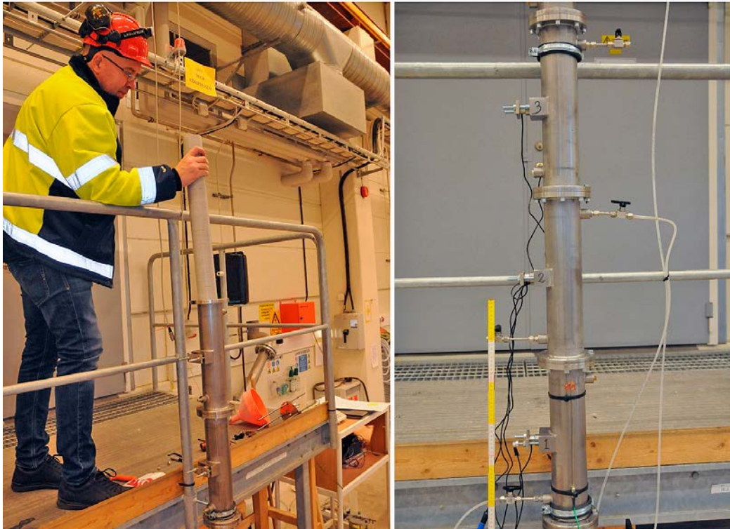
Figure 8-7. Left: Installation of one of the bentonite packages. Right: Three sensors (left side of the tube) are registering the radial swelling pressure from the bentonite section.
