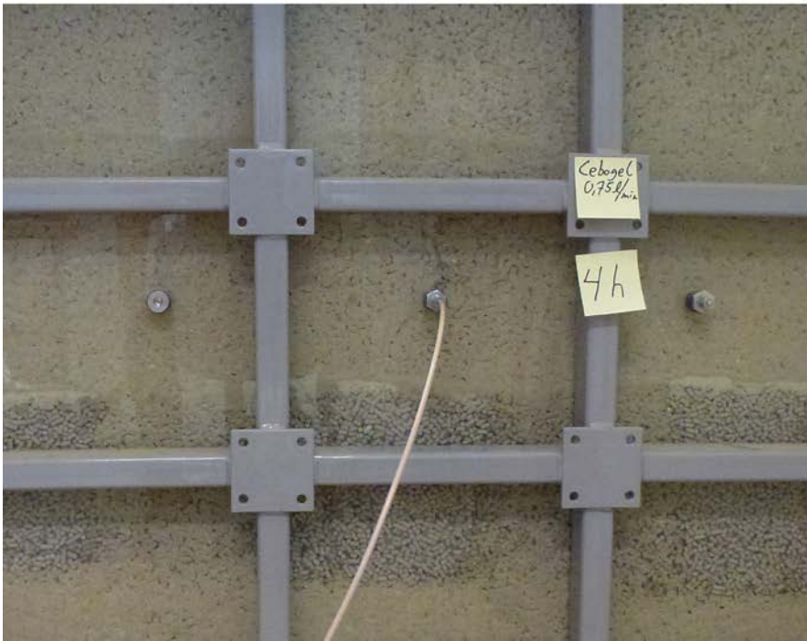
Figure 4-24. Photos showing close-ups of the test performed with layers, CL_0.75_L (Cebogel, 0.75 l/min, fines in layers). Upper: After installation Lower: At termination.
