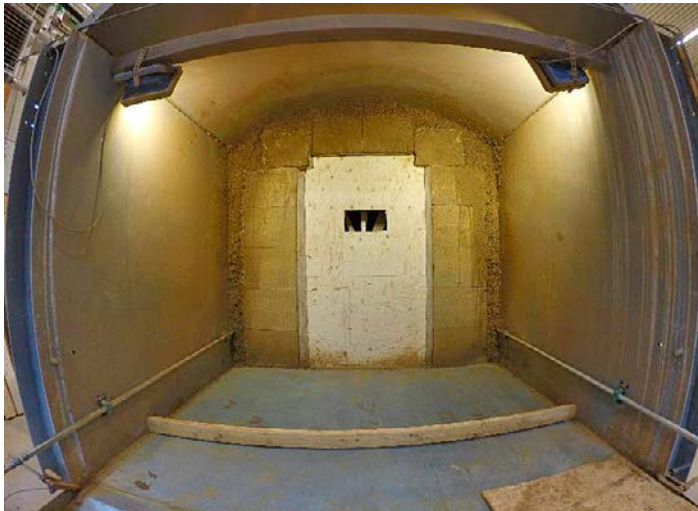
Figure 4-36. Photo showing the backfill front in Test 5 after having finished the installation.
