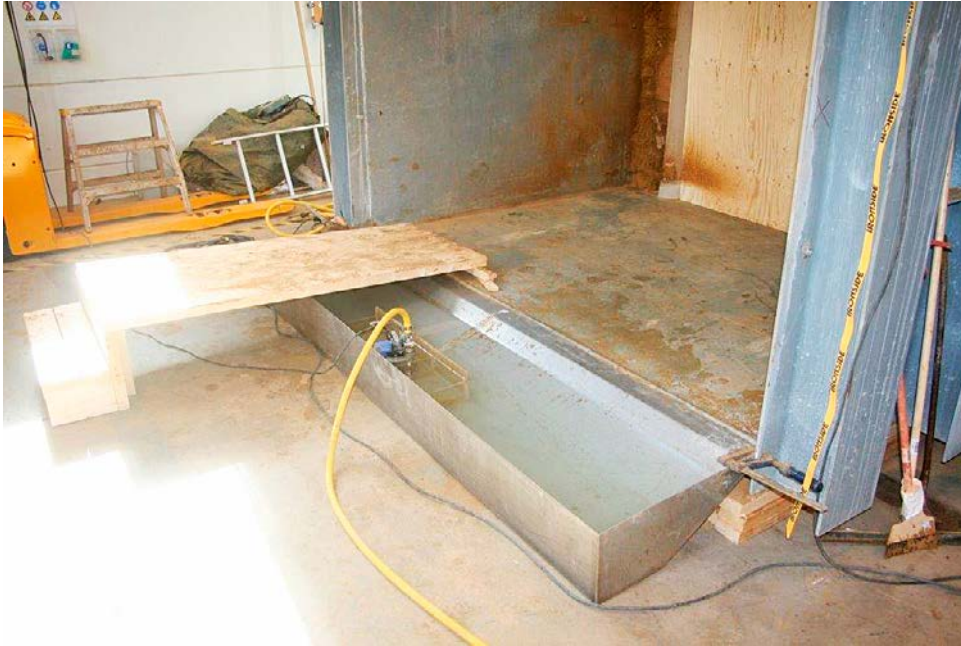
Figure 4-4. Photo showing the tray located in front of the steel tunnel.
