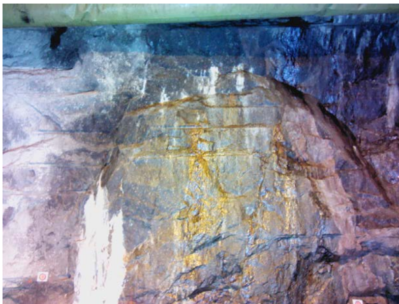
Figure 2-2. Picture #1914, Location 70Lb.
