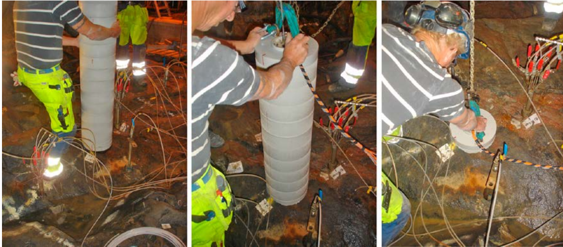
Figure 7-11. Installation of bentonite parcel in Hole 17.
