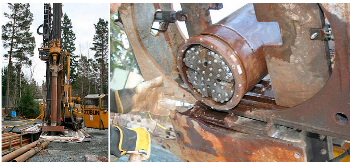
Figure 3-1. To the left the Commacchio percussion rig seen on the drill site. To the right the NO-X 280 casing is prepared for drilling through the overburden.
