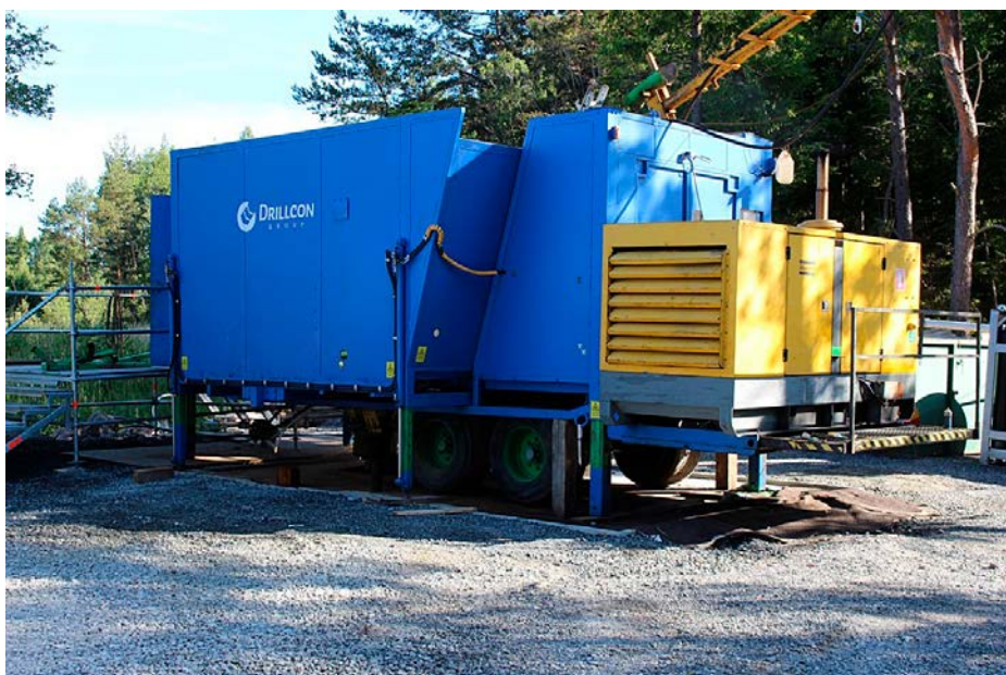
Figure 3-4. Drilling rig Boyles B20 APC.
