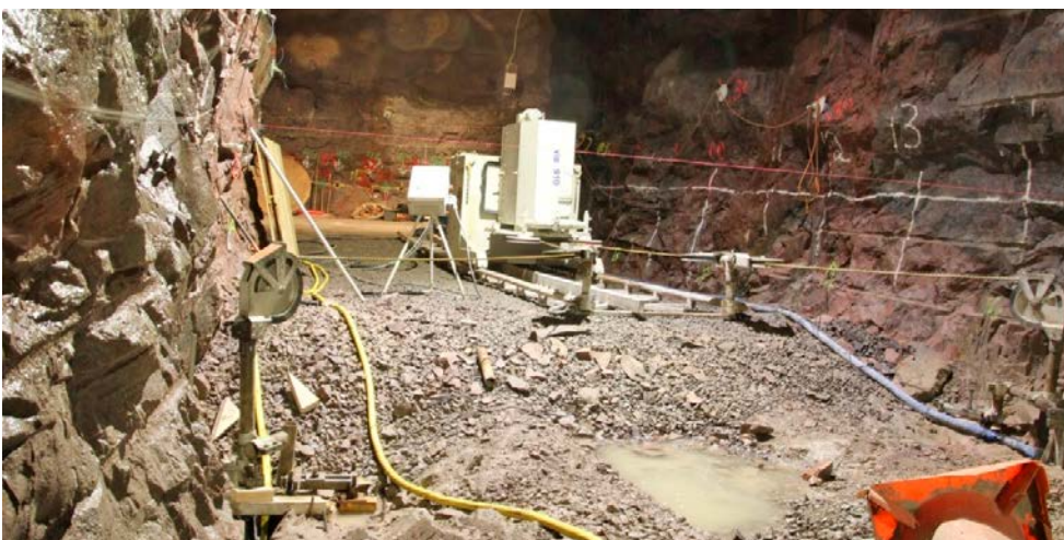
Figure 3-5. Ongoing wire sawing in TAS04 (Photo by Rickard Enér).
