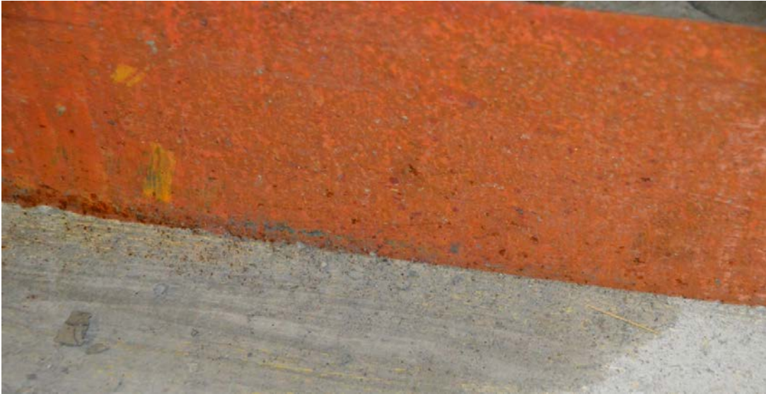
Figure 4-34. The interface between the copper joint seal and the concrete.
