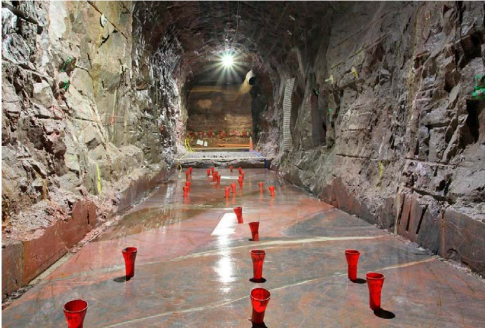
Figure 3-6. Results from wire sawing in TAS04 (Photo by Rickard Enér).
