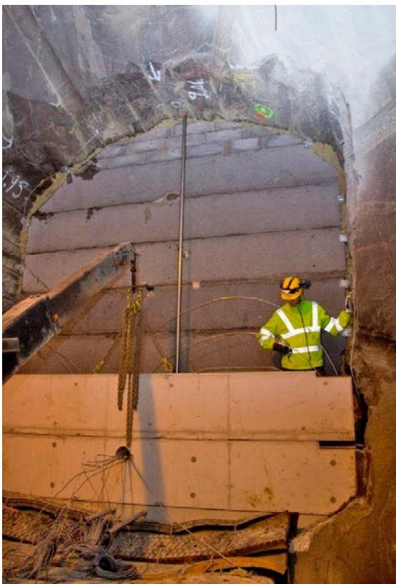
Figure 4-23. Installation of concrete beams, bentonite seal, gravel filter and sensors.
