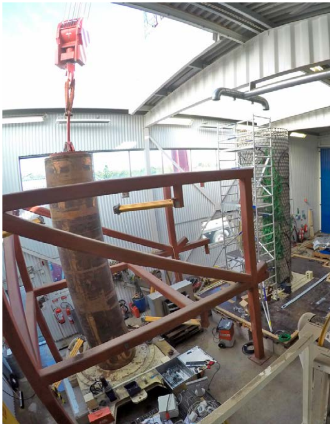
Figure 4-8. Pre-heated canister being prepared for installation inside the Supercontainer.
