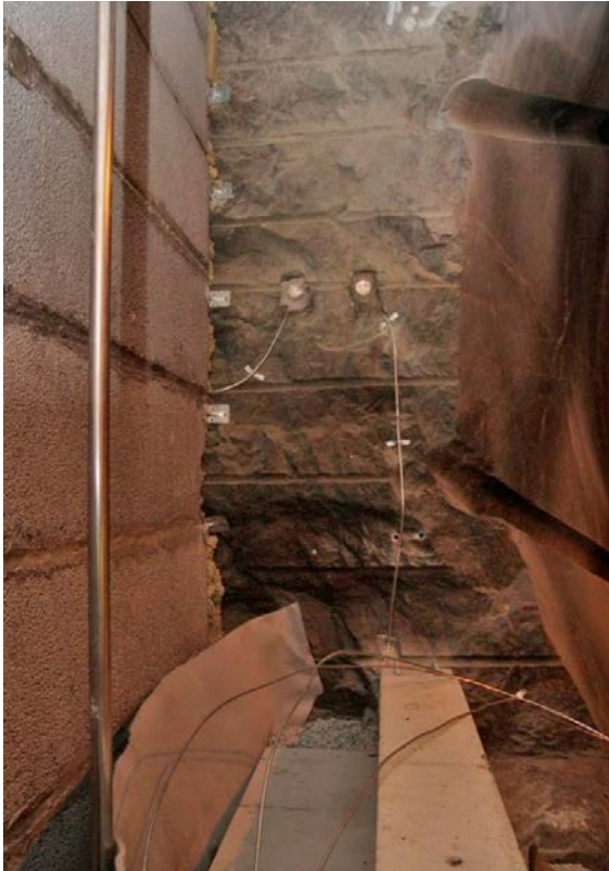
Figure 4-22. Detail photo showing (from left) delimiter of leca-beams, gravel filter with drainage (air) pipe, delimiter of geotextile, bentonite seal of MX-80 (blocks and pellets) and delimiter of concrete beams. All sensor cables are led in steel tubes.
