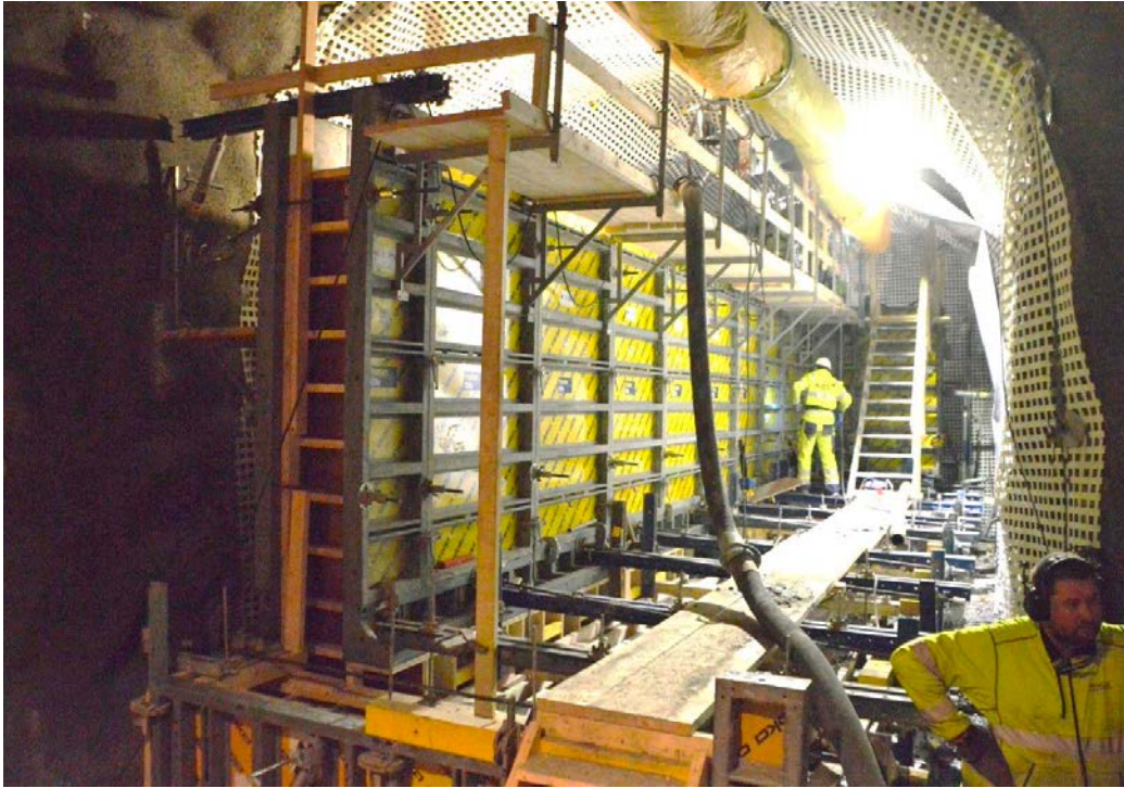
Figure 4-32. The formwork is ready.
