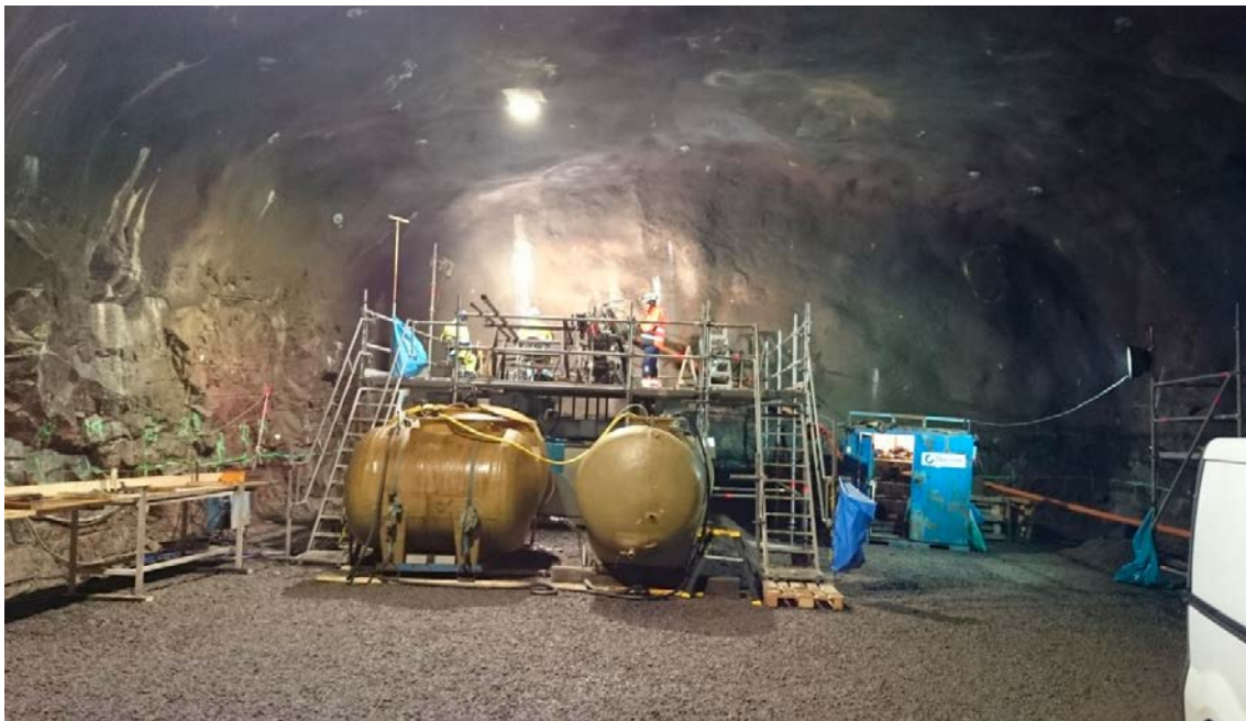
Figure 7-7. The complete drill site for borehole K08028F01 in TAS08 in operation. The drillers are working on the left side while other technician's workspace is to the right. Flush watering (tracer marked) is supplied from the two tanks in front of the platform, and a bench for retrieval of drill core from the core barrel is seen to the left. Return water from the borehole is lead to the Äspö HRL drainage system after sedimentation.
