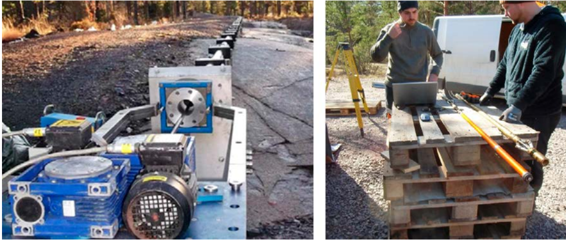
Figure 4-4. To the left, an electrically powered insertion rig is used for in and out transportation of the deviation tools in the 300 m long plastic tube. To the right Devico technicians prepare some of their instruments before measurement.
