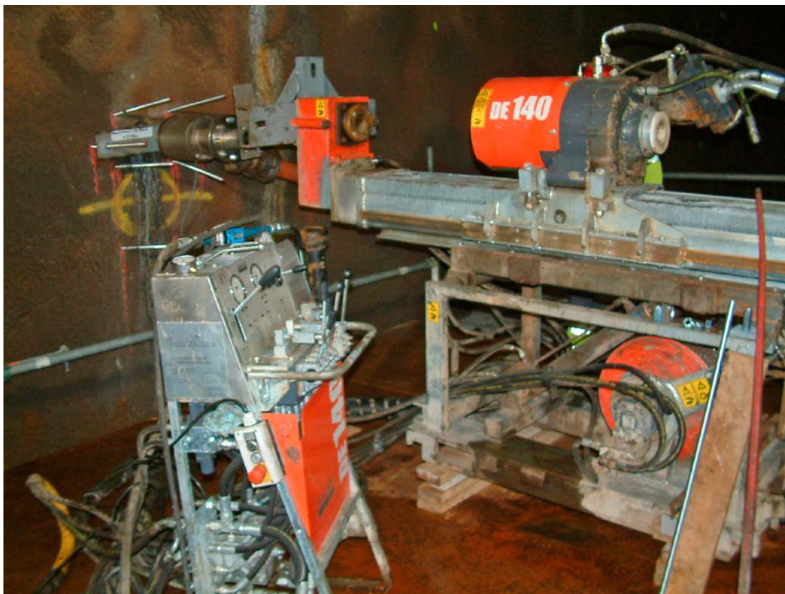
Figure 7-8. The drilling rig Sandvik DE140 was used for drilling of K08028F01.
