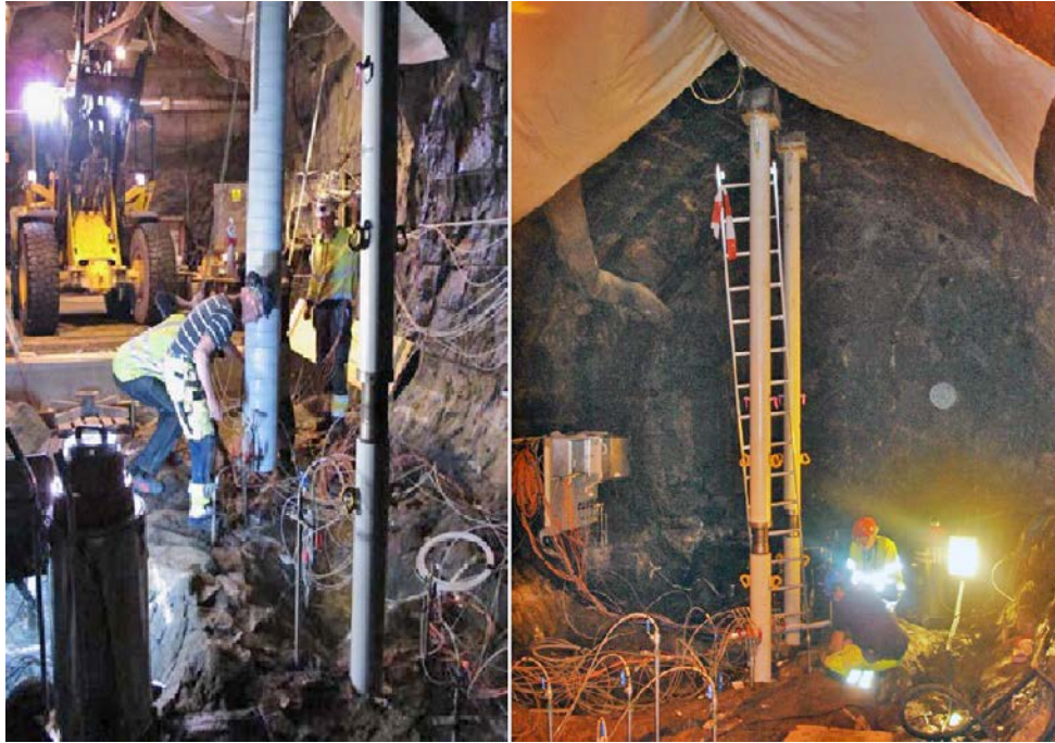
Figure 4-11. Pillars between bentonite parcels and roof.
