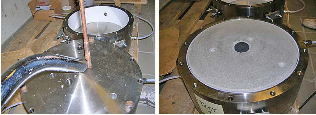
Figure F-7. Drilling of holes for RH-sensor holders.
