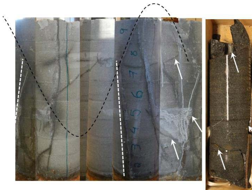
Figure 5-16. Comparison of some fractures in rock core and traces on bentonite for KO0017G01. Black dashed line approximate location of main fracture and white dashed line approximate location of pegmatite vein.
