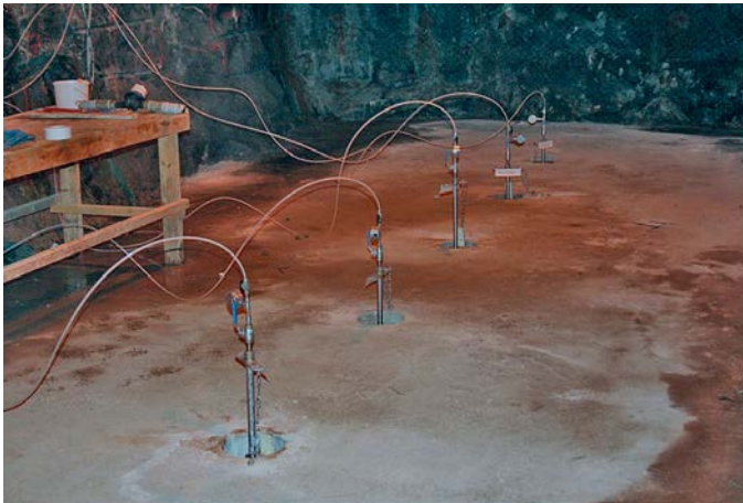
Figure 3-3. TASO-tunnel (Phase 1) and the five boreholes (borehole distance 1.5 m) used for initial characterisation and selection of site. Picture includes the packers and the concrete slab.
