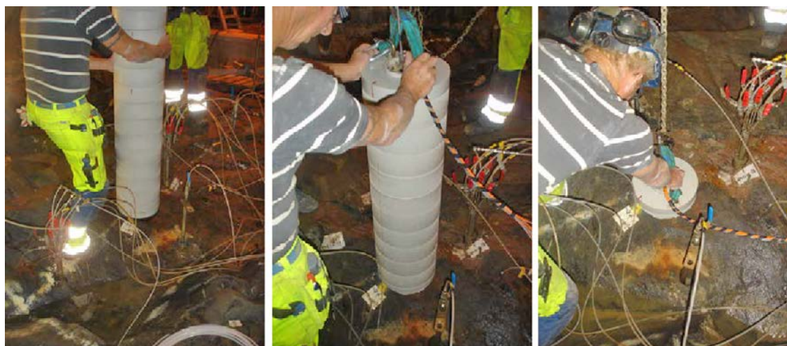
Figure 4-10. Installation of bentonite parcel in Hole 17.
