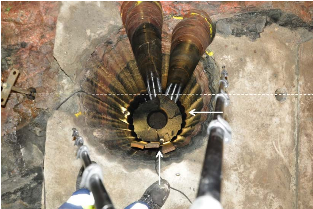
Figure 5-21. Borehole KO0018G01 following stitch drilling and dismantling. New (not previously identified) fractures being more or less parallel or perpendicular to tunnel (indicated by dashed, white line) and close to in line with adjacent boreholes.
