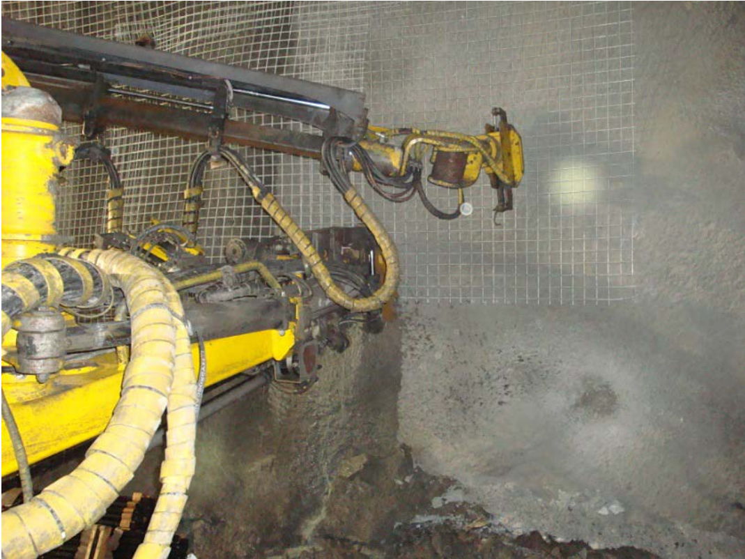
Figure 7-2. Installation of welded wire mesh with an Atlas Copco Boltec rig.
