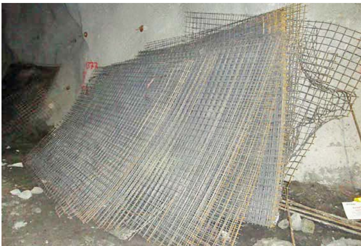
Figure 7-5. Sections of welded wire mesh.
