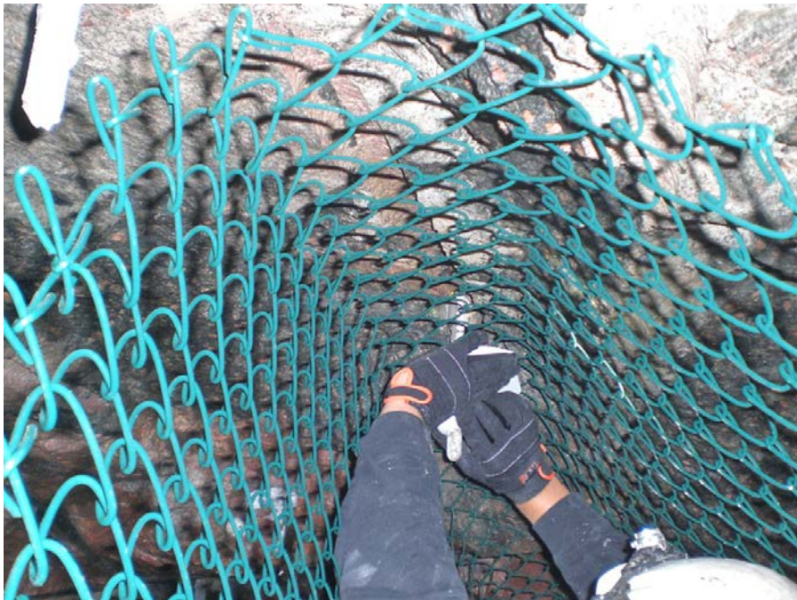
Figure 6-4. Hand installation of chain linked wire mesh in TASS.
