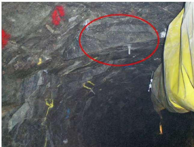
Figure 3-7. Example of geometry deviation in the end of a blast round. Note the bolted block in the beginning of the next round.
