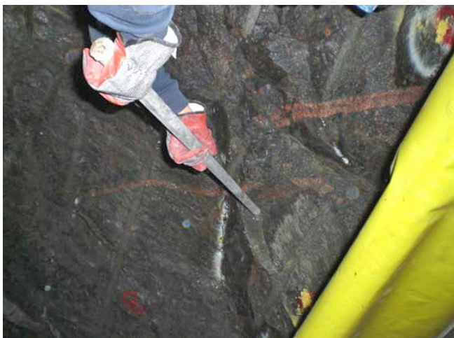
Figure 5-2. Hand scaling in TASS.
