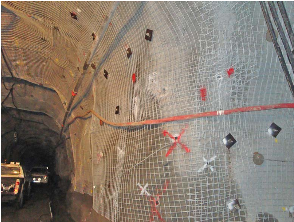
Figure 7-1. Dynamic reinforcement in the Kiruna mine.
