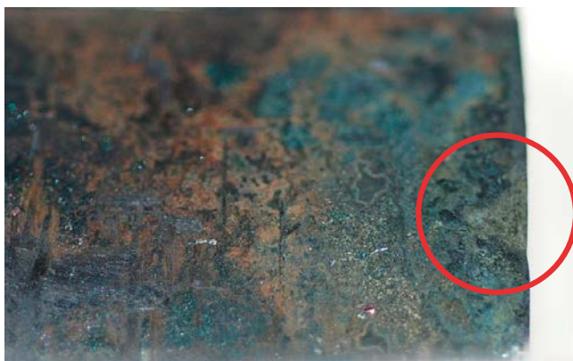
Figure 4-59. Cast iron insert sample M5 30:1 inside its sample holder with the corroded area encircled.
