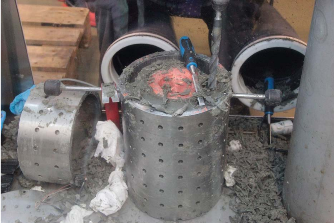
Figure 2-12. Removal of bentonite at the bottom of the A05 support cage from MiniCan to expose the copper canister.
