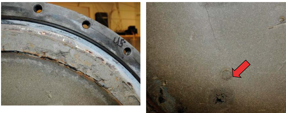
Figure 4-13. BB IV, cross section A. LEFT: Close up showing the bentonite filled SC-rock gap. RIGHT: Close up showing the position of where the piston of the axial pressure measurement A2 has been in contact with the bentonite block surface. A sample was taken at this position.
