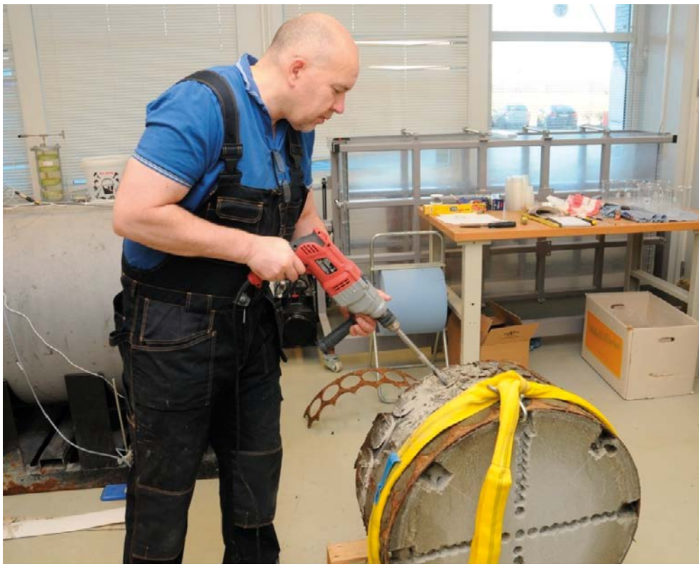
Figure 4-24. BB IV, cross section B. In order to uncover cross section B inside the SC the bentonite was removed by using a combination of seam drilling and sawing.
