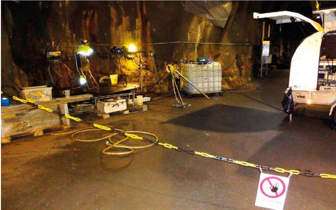
Figure 5-2. Measuring trailer mobilised at K03009F01.
