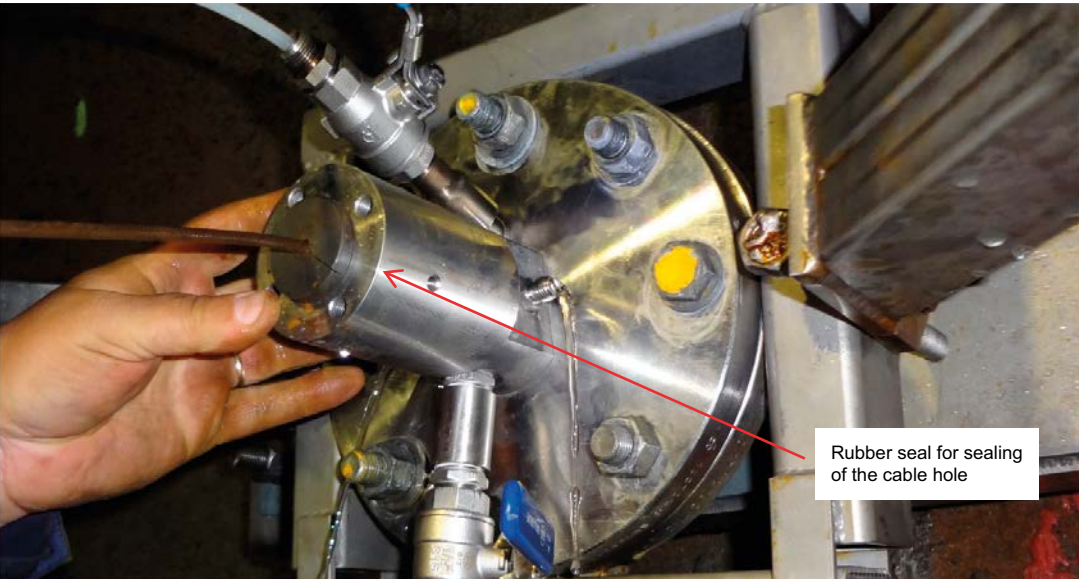
Figure 5-5. The sealing unit attached to a borehole casing.
