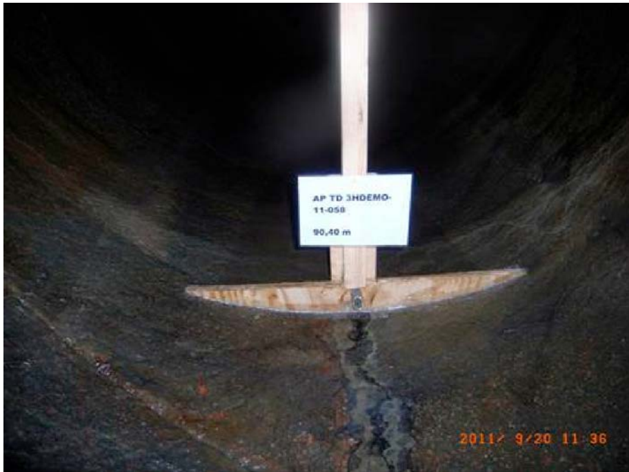
Figure 7-3. Wooden weir used to enable monitoring of groundwater inflow into the MPT drift.
