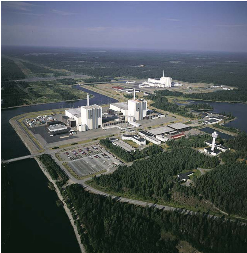
Figure 16-3. The Forsmark power station with the three BWR reactors F1, F2 and F3 from left to right in the picture.
