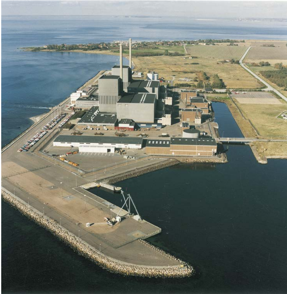
Figure 15-1. View of the Barsebäck NPP with the two BWR reactors B1 (closest in the picture) and B2.
