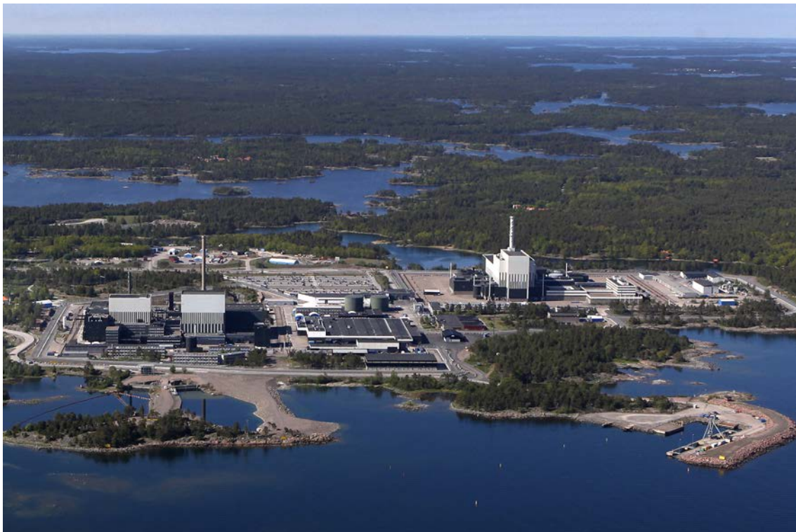
Figure 15-3. OKG nuclear power plant with the three BWR reactors O1, O2 and O3 from left to right in the picture.
