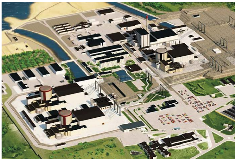
Figure 16-1. Ringhals NPP with reactors 1 and 2 to the right and reactors 3 and 4 to the left. In the centre of the site, there are for example office buildings and a lunch restaurant. Just above R1 in the image is the plant's area for handling, conditioning and storage of radioactive waste.
