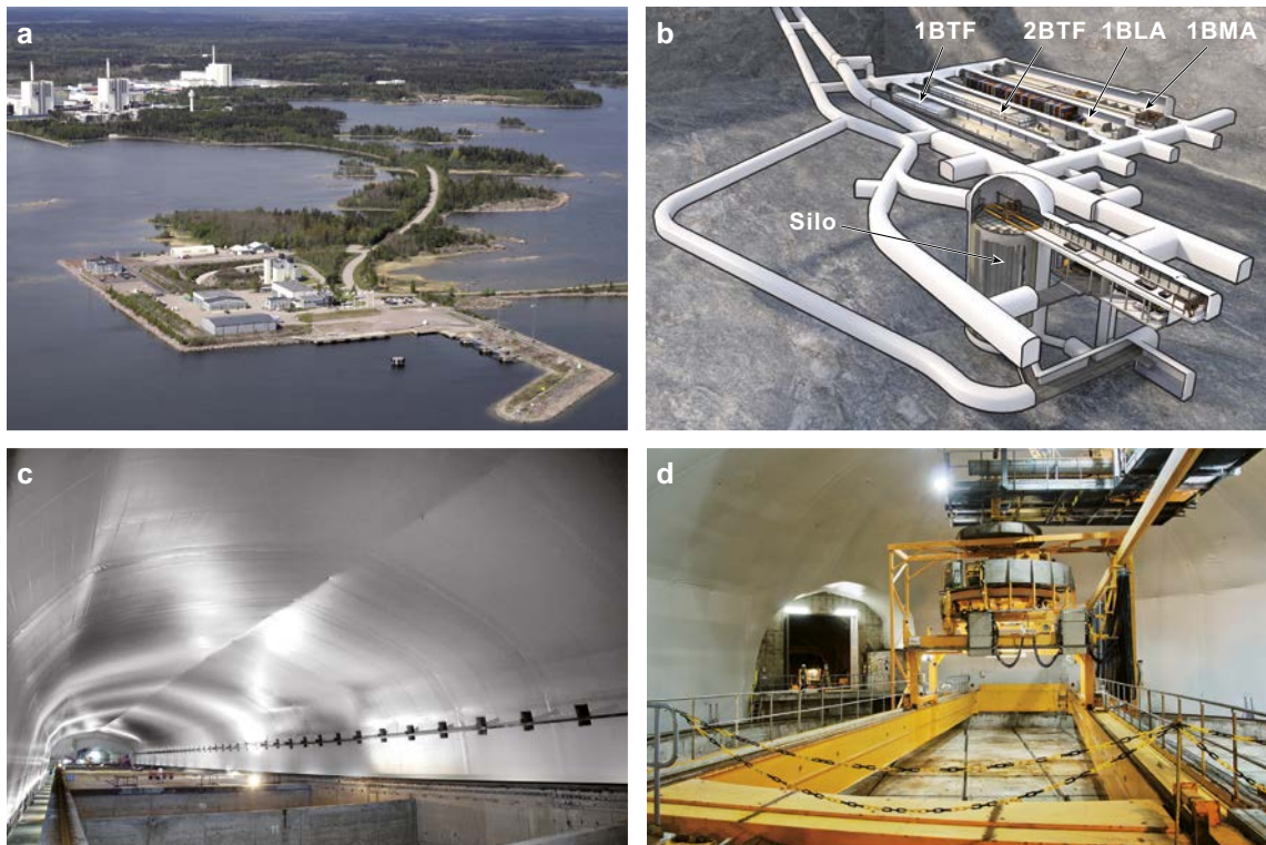
Figure 2-2. The final repository for short-lived radioactive waste, SFR consists of two rock vaults for concrete tanks (1–2BTF), one waste vault for low-level waste (1BLA), one waste vault for intermediate-level waste (1BMA) and a silo for intermediate-level waste a) View of the surface facility, b) SFR underground, c) Rock vault, d) View of the silo top.
