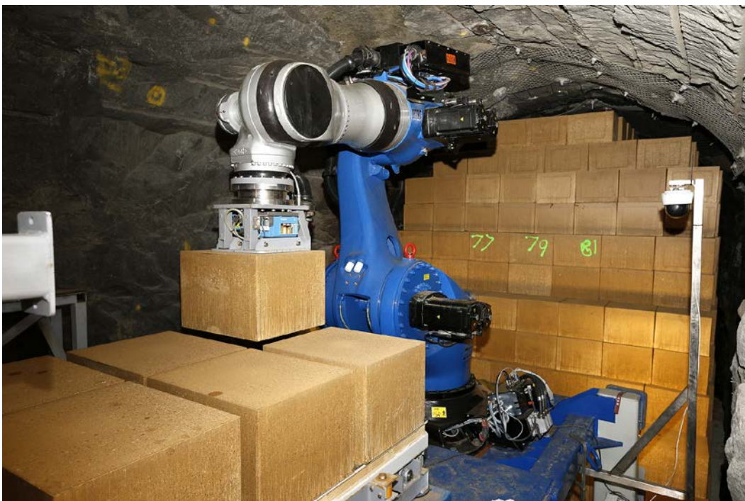
Figure 10-19. Block installation at 450 metres depth in the Äspö HRL.
