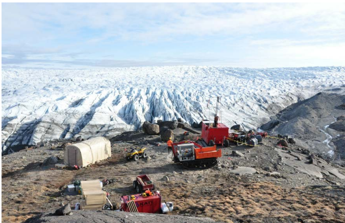
Figure 5-5. Drilling of DH-GAP04. The site was selected as close to the ice margin as possible in terms of safety and logistics. Photo from June 2011, by Anne Lehtinen.
