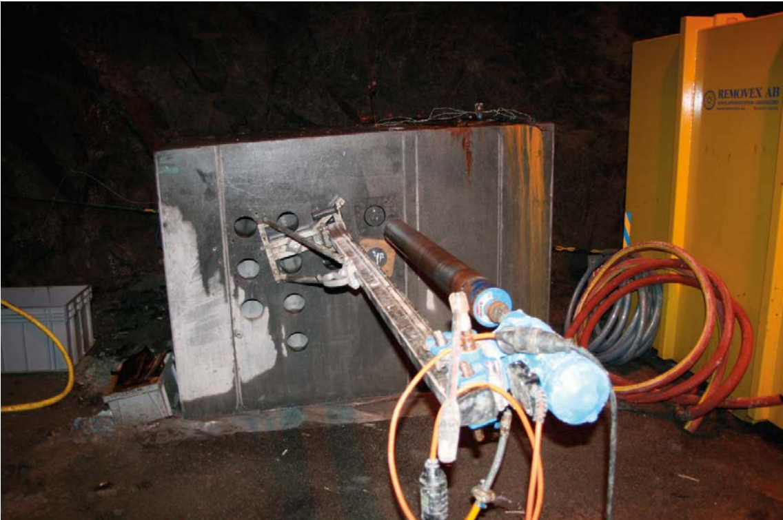
Figure 4-24. Cores being taken out of the monolith.
