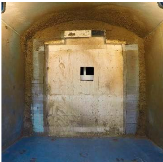
Figure 4-26. Photo showing Test 3 after installation of backfill including the concluding vertical pellet wall.
