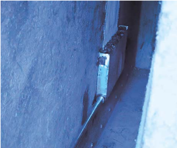
Figure 4-28. Mounting of water collector prototype in the steel tunnel.
