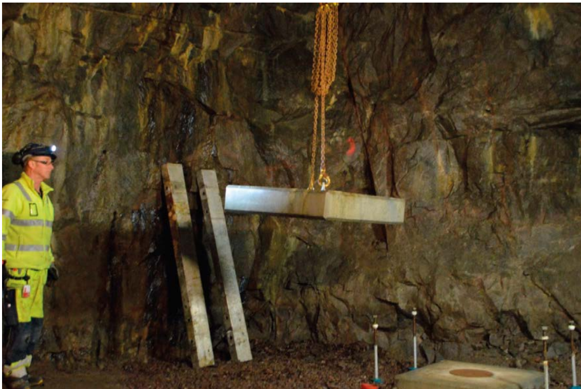
Figure 4-18. The lid is removed from the deposition hole.
