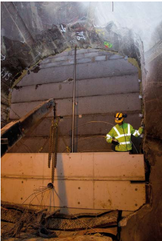
Figure 4-35. Installation of concrete beams, bentonite seal, gravel filter and sensors.
