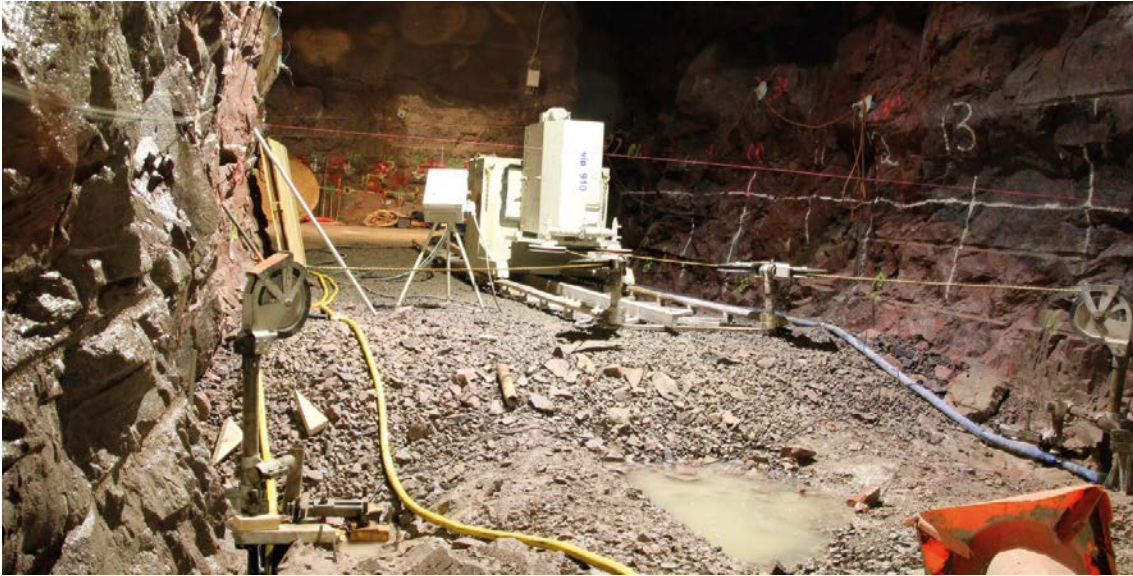
Figure 4-46. Ongoing wire sawing in TAS04 (Photo by Rickard Enér).
