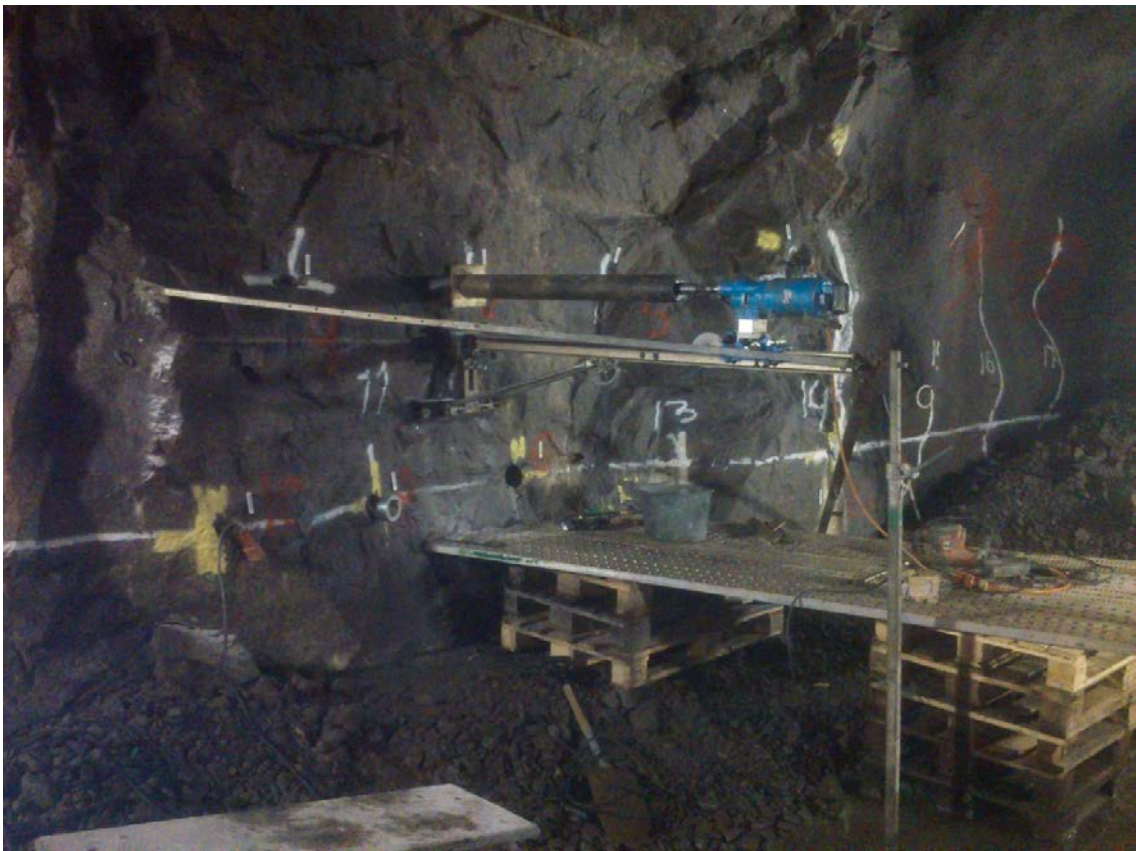
Figure 4-22. Overcoring of bolts for investigation.
