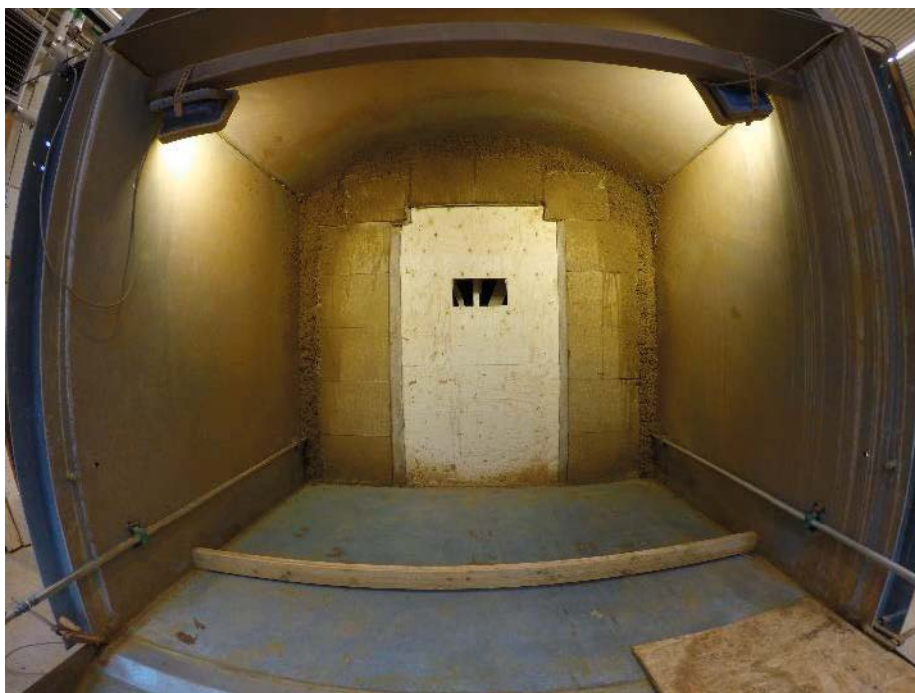
Figure 4-30. Photo showing the backfill front in Test 5 after having finished the installation. The two drainage pipes can be seen on each wall leading out from the tunnel.
