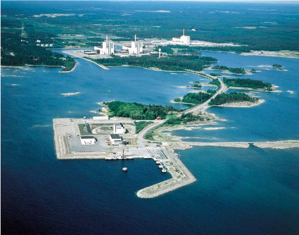
Figure 1-2. The surface part of the SFR facility in the Forsmark harbour with the nuclear power plant in the background.
