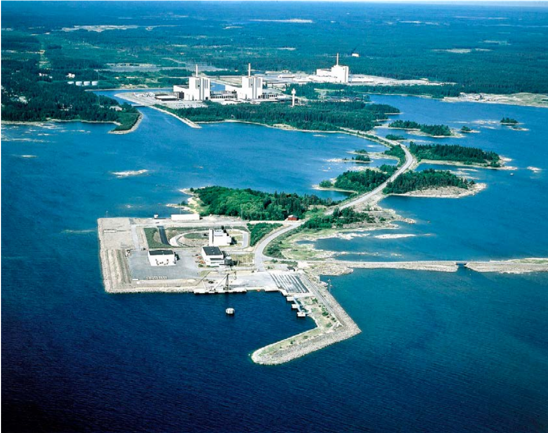
Figure 1-1. The surface part of the SFR facility in Forsmark harbour with the Forsmark nuclear power plant in the background.
