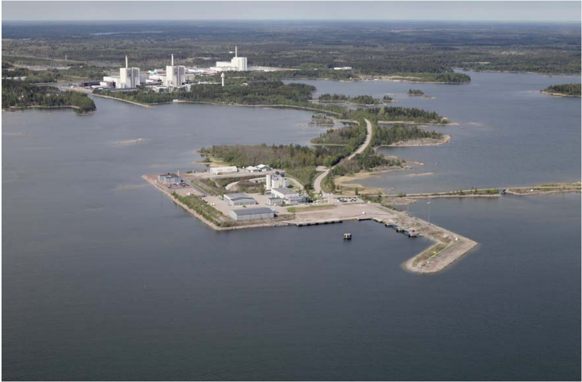
Figure 1-2. The surface facilities of SFR 1 in the Forsmark harbour. The subsurface parts of SFR 1 are located beneath the sea floor, approximately 700 m from the surface facilities.
