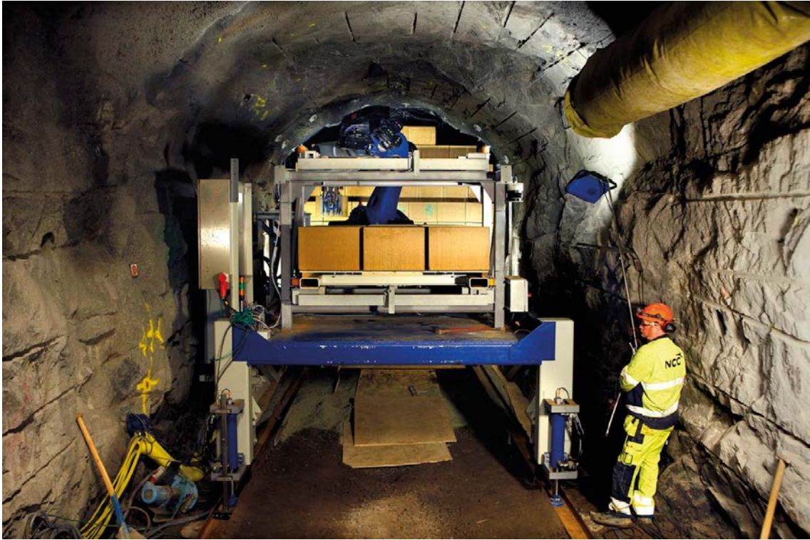
Figure 8-5. Robot platform with block feeding system and installation robot.
