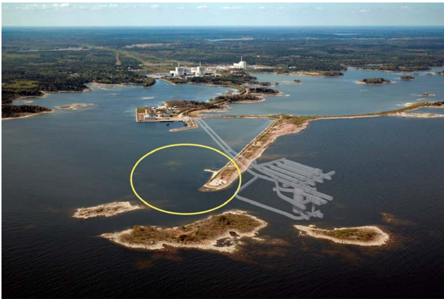
Figure 1-3. Figure showing the existing SFR facility (SFR 1) and the suggested area (yellow) for the SFR extension (SFR 3) in the foreground and the Forsmark nuclear power plant buildings in the background. The distance from SFR 1 to the shoreline is about 2 km. The man-made wave breaker running above SFR 1 is referred to as the 'SFR Pier', cf. Figure 1-1.
