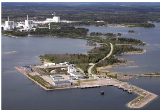
Aerial view of the surface part
