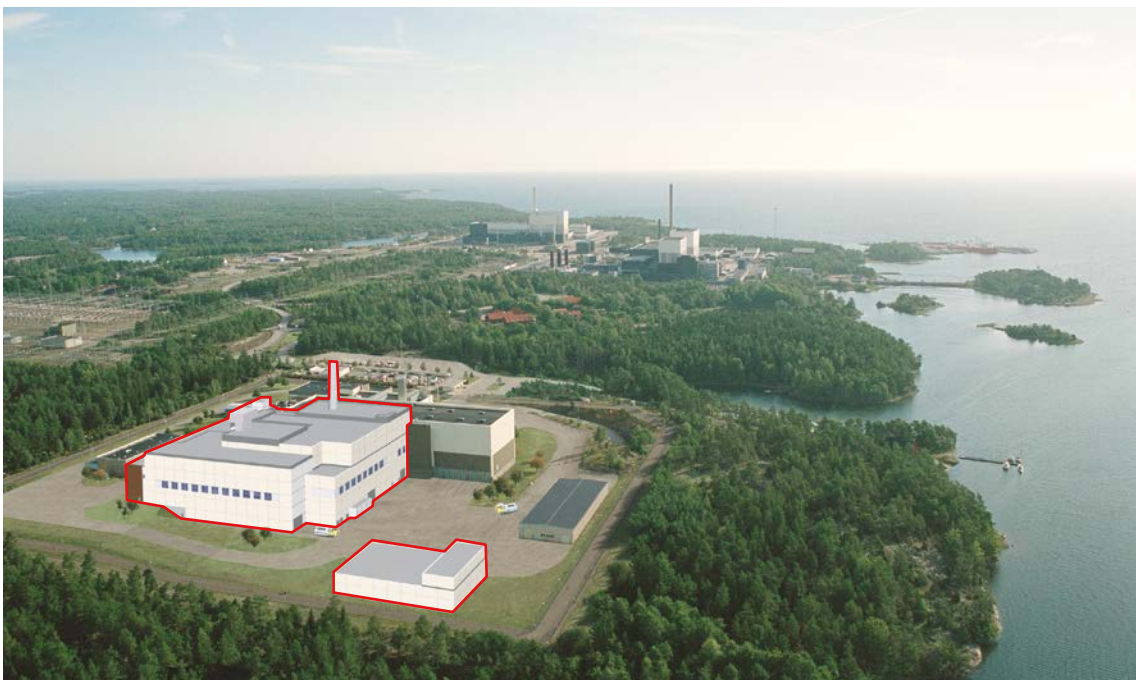
Figure 3-11. Clink with encapsulation section for spent nuclear fuel (marked in the figure).
