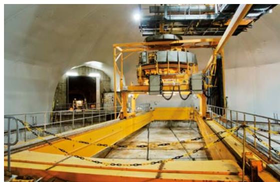
View over top of silo
