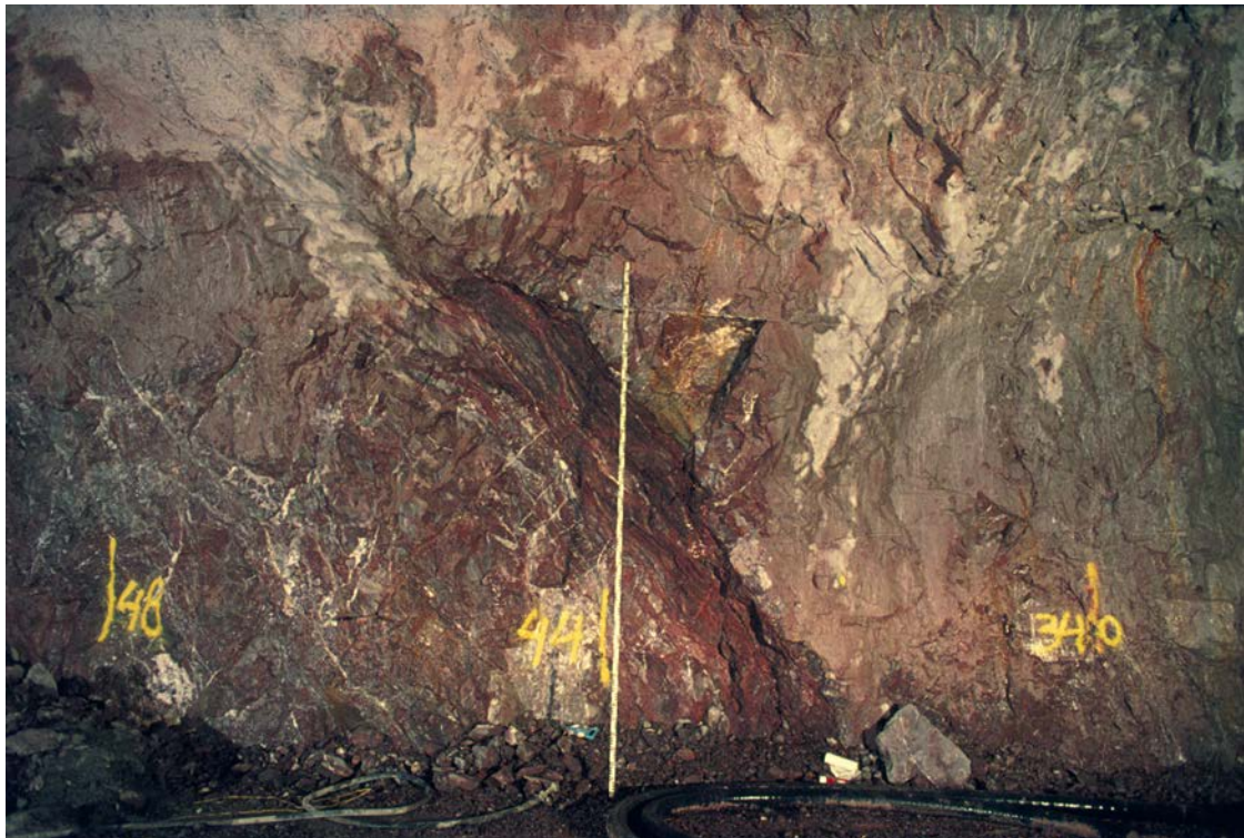
Figure A-1. Clay-filled fracture in brecciated metagranite within the Singö Deformation Zone, Forsmark 1 and 2 tunnel (Carlsson and Olsson 1977, Carlsson and Christiansson 2007, Figure 4-3).
