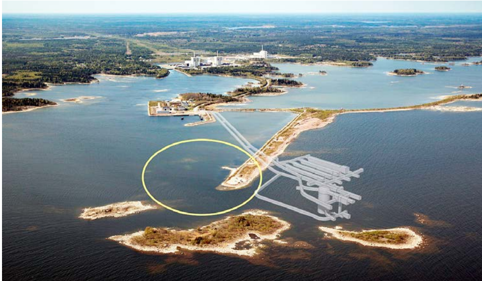
Figure 1-3. Figure showing the existing SFR facility (SFR 1) and the suggested area (yellow) for the SFR extension (SFR 3) in the foreground and the Forsmark nuclear power plant buildings in the background. The distance from SFR 1 to the shoreline is about 2 km. The strip of land (a man made wave breaker) running above the SFR 1 tunnels is referred to as the 'SFR Pier' in this report, cf. Figure 1-1.
