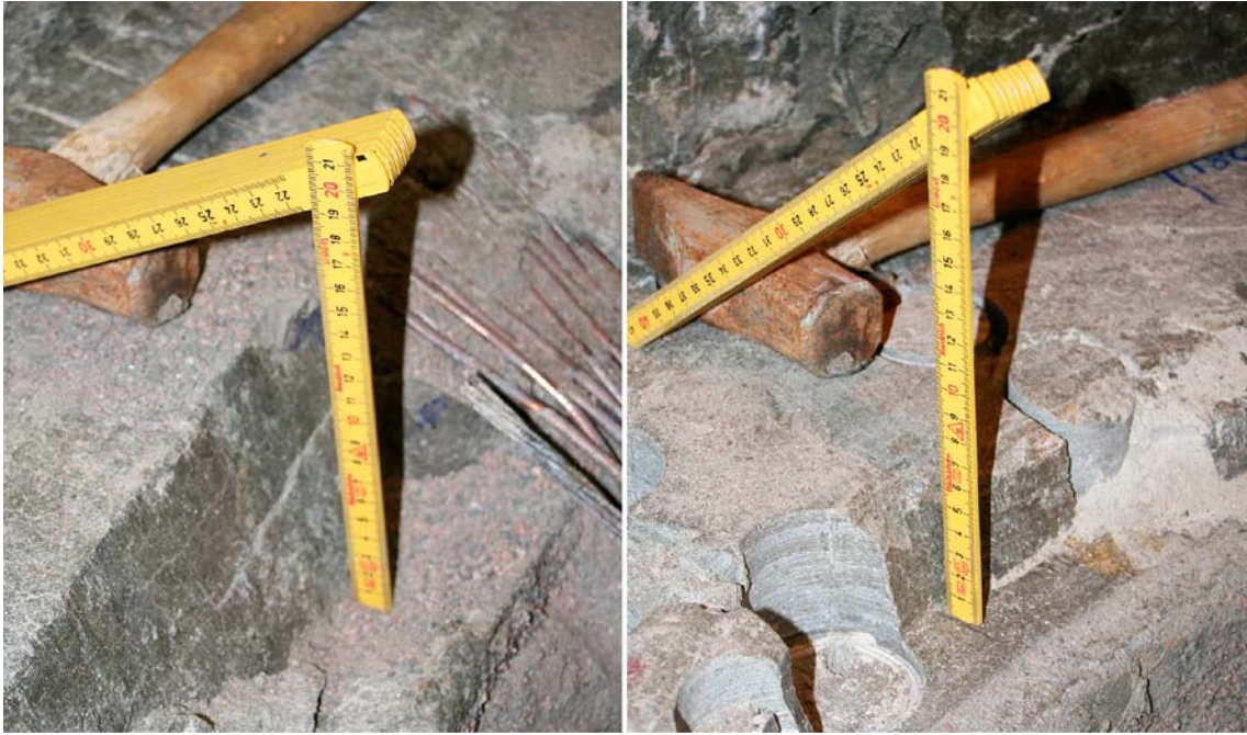
Figure 4-2. Shelves of top surface of Ring 12 indicating shearing. Left: in 350° direction inclination approximately 65° in relation to the horizontal plane; right: in 200° direction inclination approximately 72° in relation to the horizontal plane.
