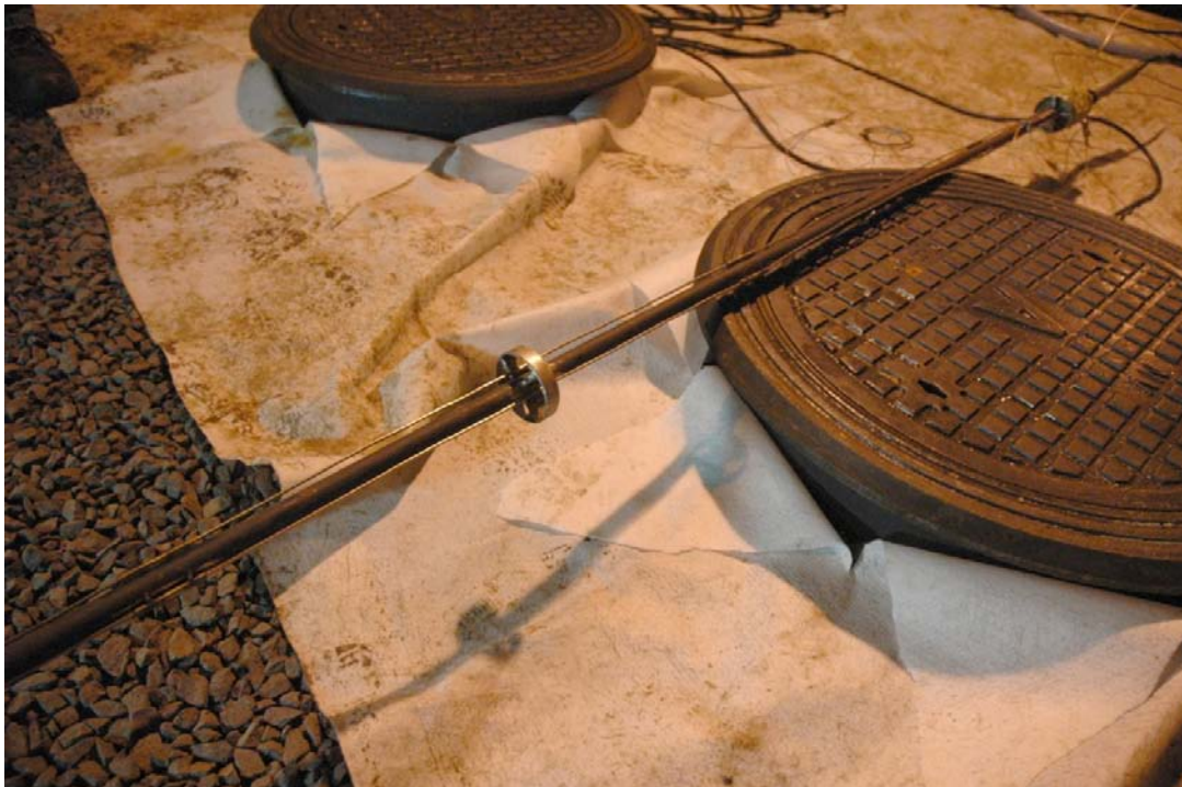
Figure 3-11. The heater equipment used for heating in the SLITS pilot test borehole. The length of the heater is 4 m. The heater is kept centred with three holders with the diameter of the borehole, 76 mm.
