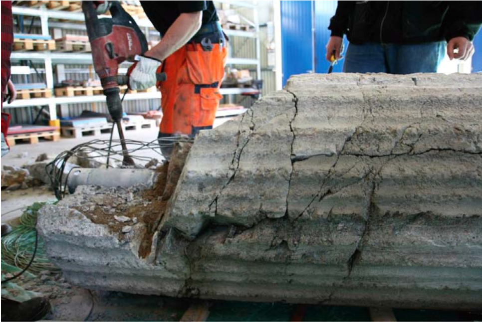
Figure 5-8. Parts of the rock cover was rather fractured.
