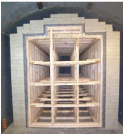
Clay Block Assembly prior to pellet installation
