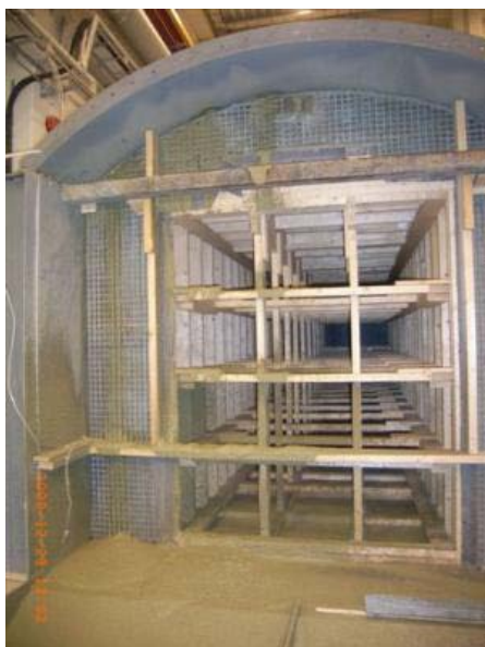
Outflow at crown
