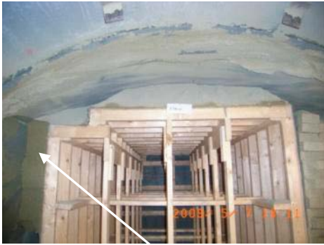
Flow path for water at upper left (Dark feature)
