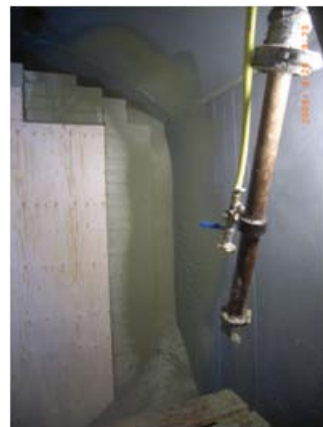
Installing clay pellets showing spray nozzle (foreground)
