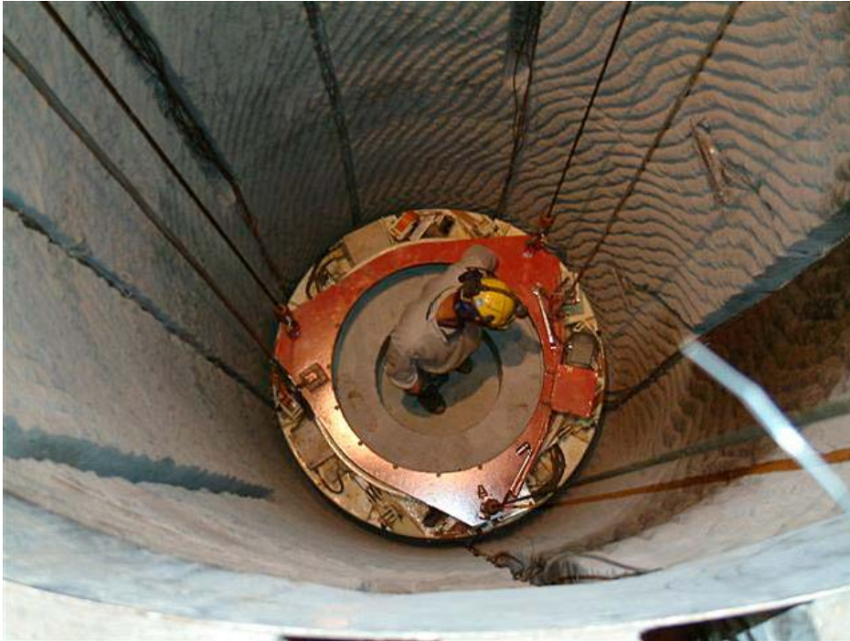
Figure 8-2. The first block placed at the bottom of the deposition hole.
