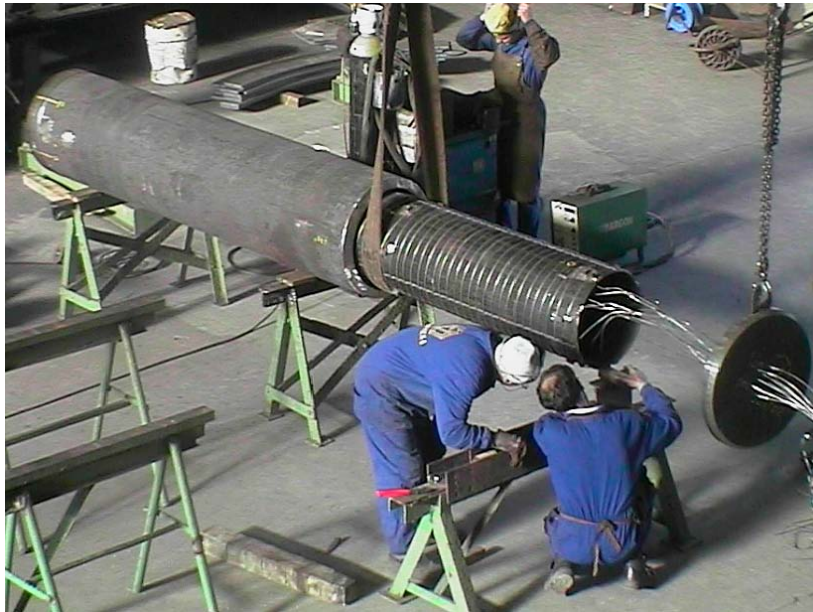
Figure A4-7. Heater construction: external case, inner tube with heating elements wound up and lid with passthroughs.
