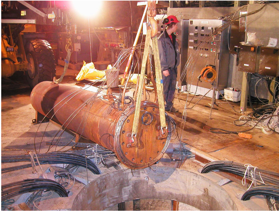
Figure 8-3. The heater just before it is placed in the deposition hole.
