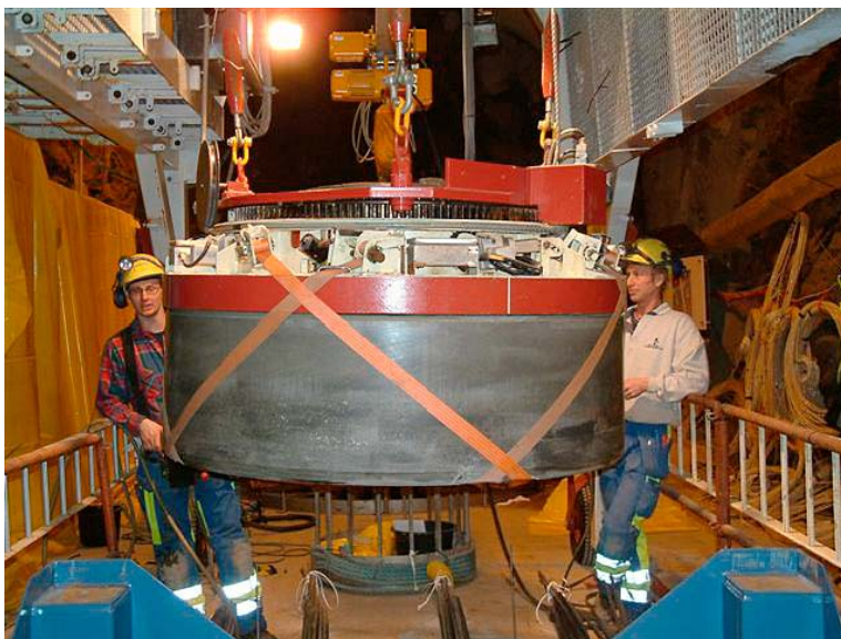
Figure 8-1. A bentonite block attached to the lifting equipment with four straps.
