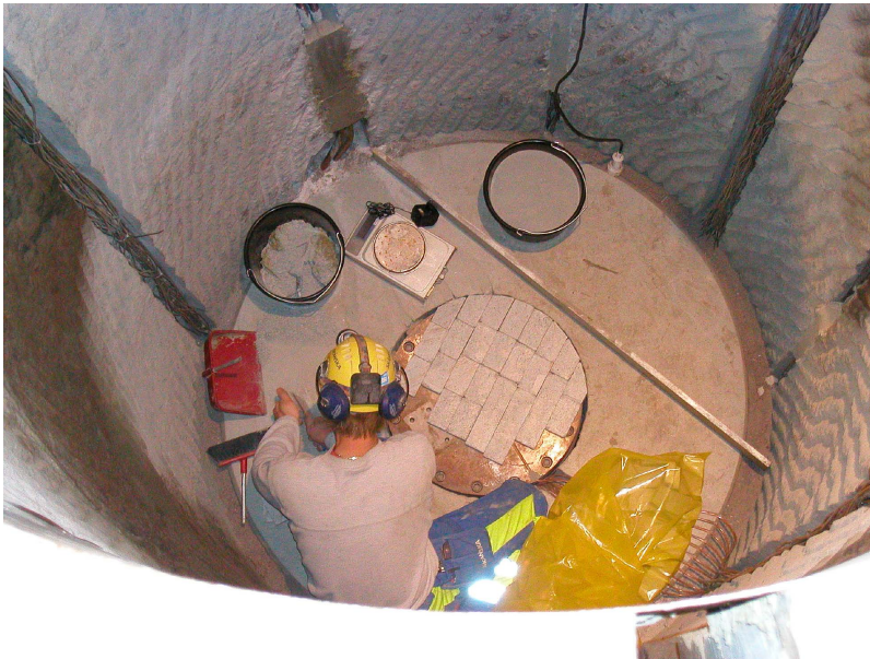
Figure 8-5. Small bricks of bentonite are placed on top of Heater 1.
