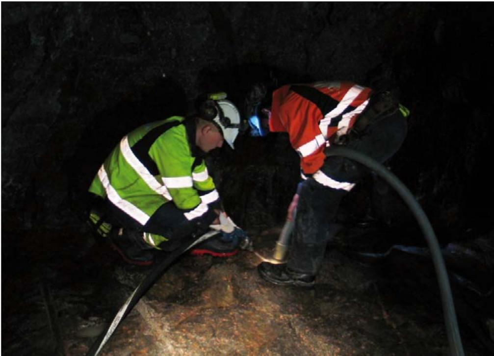
*Figure 2-5. Cleaning the tunnel floor with the help of water and an industrial vacuum cleaner somewhere within section 21–48 m.*
