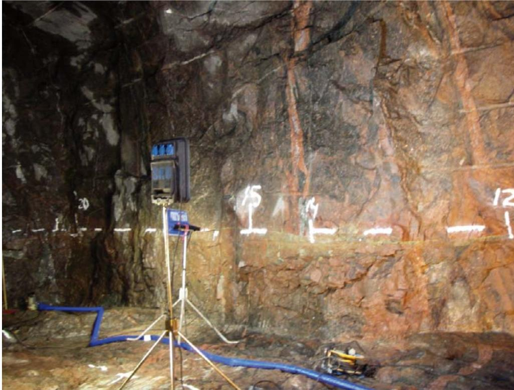
*Figure 2-6. Floodlights illuminating the TASS-tunnel, section 12–20 m. The figure also shows the painted white line marking on a level 1 m above the theoretical tunnel floor and some section markings on the wall. In the lower left-hand part of the figure, part of the painted floor centre line is visible.*
