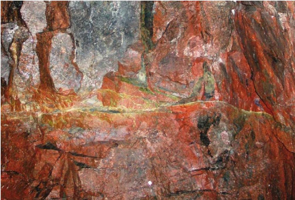
*Figure 3-16. Front, section 12.75 m, right-hand side. Sub-horizontal, epidote/prehnite-healed fracture, partly fracture network in oxidized rock, mostly Äspö diorite. Upper left-hand corner, some smooth joints.*
