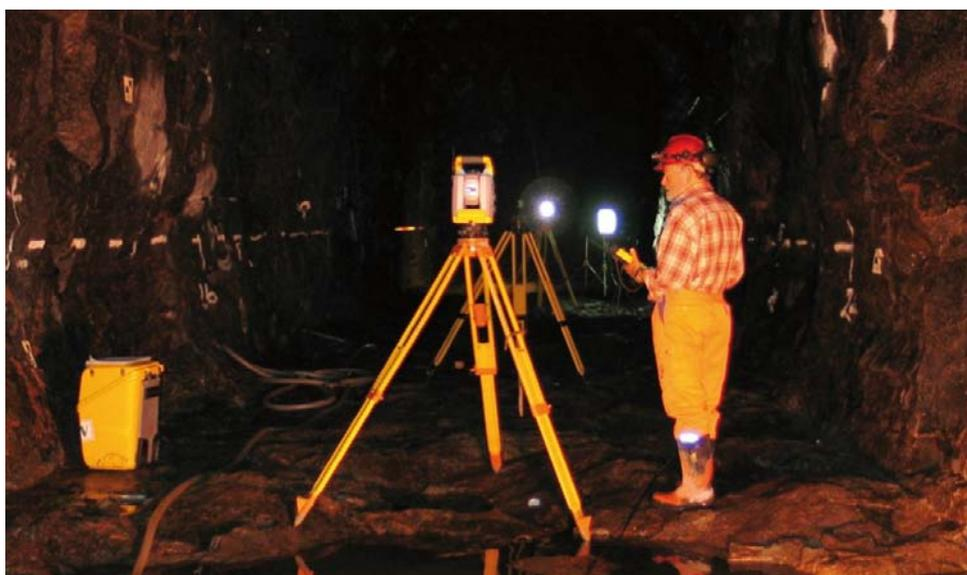
**Figure 5-2.** TASS-tunnel, section 20.7–48.7 m. Geodetic survey of complementary reference markers.
