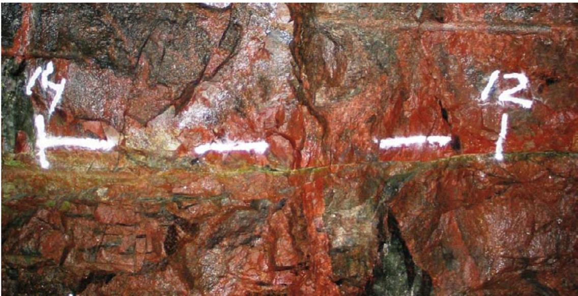
**Figure 3-32.** Right-hand wall, section 12–14 m, sub-horizontal, fracture ID: F-03 (ID comes from first full-face mapping at 8.7 m tunnel length, Appendix I), width: 5 mm, designated orientation: 000/00 (see Appendix II A). The fracture is dominated by epidote, but both prehnite and calcite also occur.
