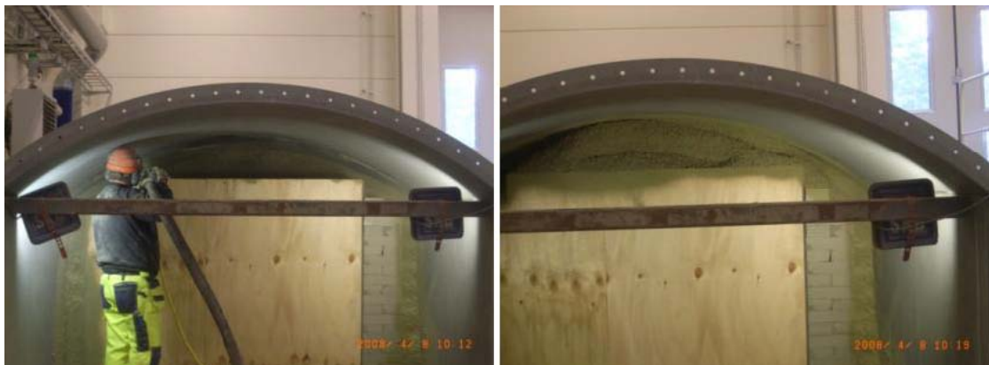
Figure 2-7. Tests to evaluate ability to place Cebogel QSE backfill pellets in 1/2-Scale tunnel simulator. (Moisture added to pellets during blowing resulting in ability to place pellets easily and in near-vertical manner.)
