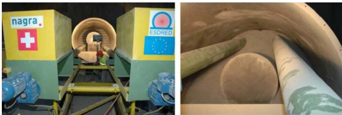
Figure 2-12. Placement trials of tunnel fill using twin-auger technique. (De Bock et al. 2008: Note NAGRA canister-sized cylinder placed in tunnel.)
