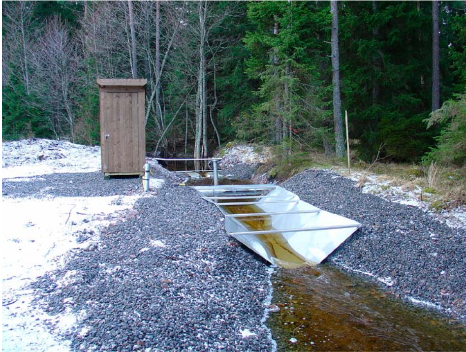
Figure 3-1. Discharge station PFM002667 with the large flume in the foreground, the small flume upstream in the background, and the service module with the LPG burner used for de-icing to the left. The tube in the middle of the brook, between the flumes, is screened and contains the devices for measurement of electrical conductivity and temperature.
