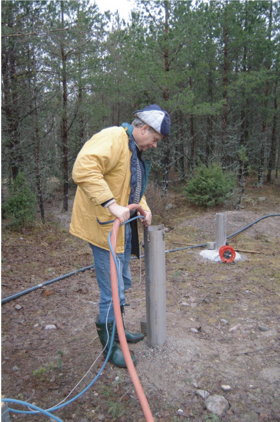
Figure 4-1. Pumping test arrangement. The red hose is used for discharge of pumped water from the pumping well SFM0061. Monitoring well SFM0060 is seen in the background.
