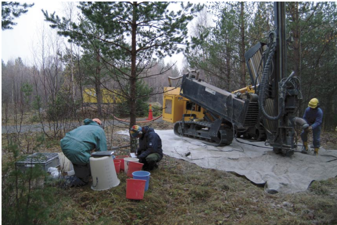
Figure 3-1. Drilling for the pumping well SFM0061 at the Börstil esker.
