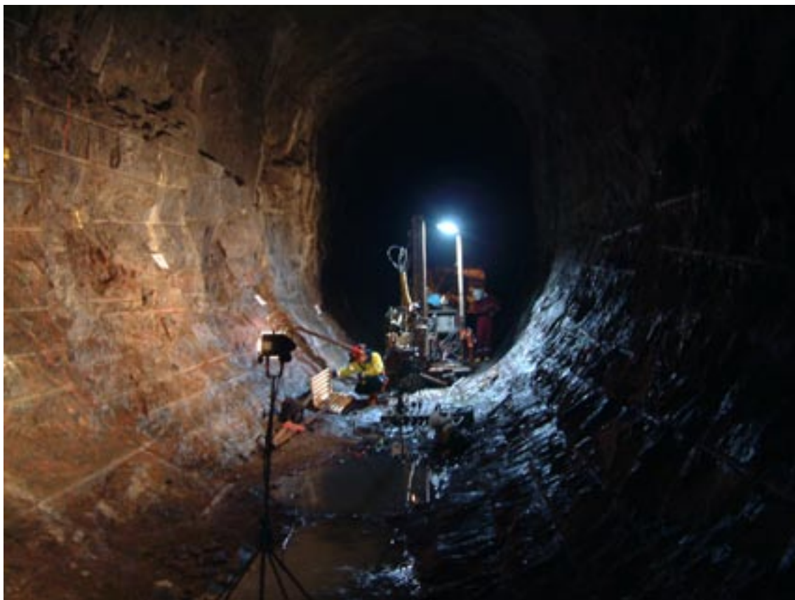
Figure 5-5. The contour of the completed APSE tunnel.
