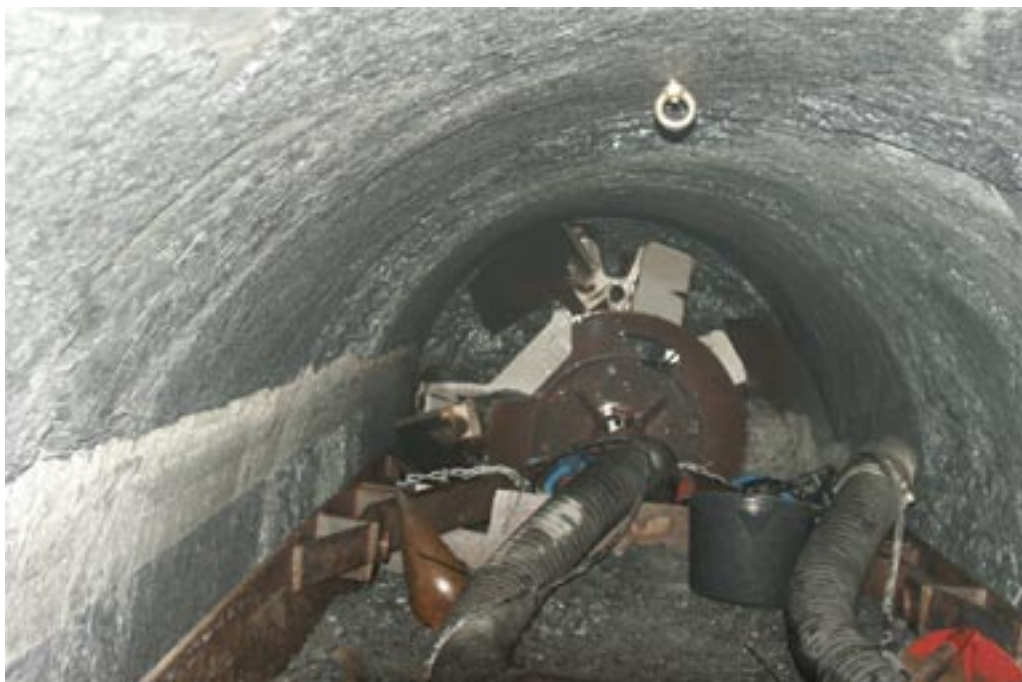
Figure 4-33. Picture from the Norwegian Sandvika project in October 2003. The photo shows the reamer from behind and the slurry system. Courtesy Atlas Copco Construction & Mining.
