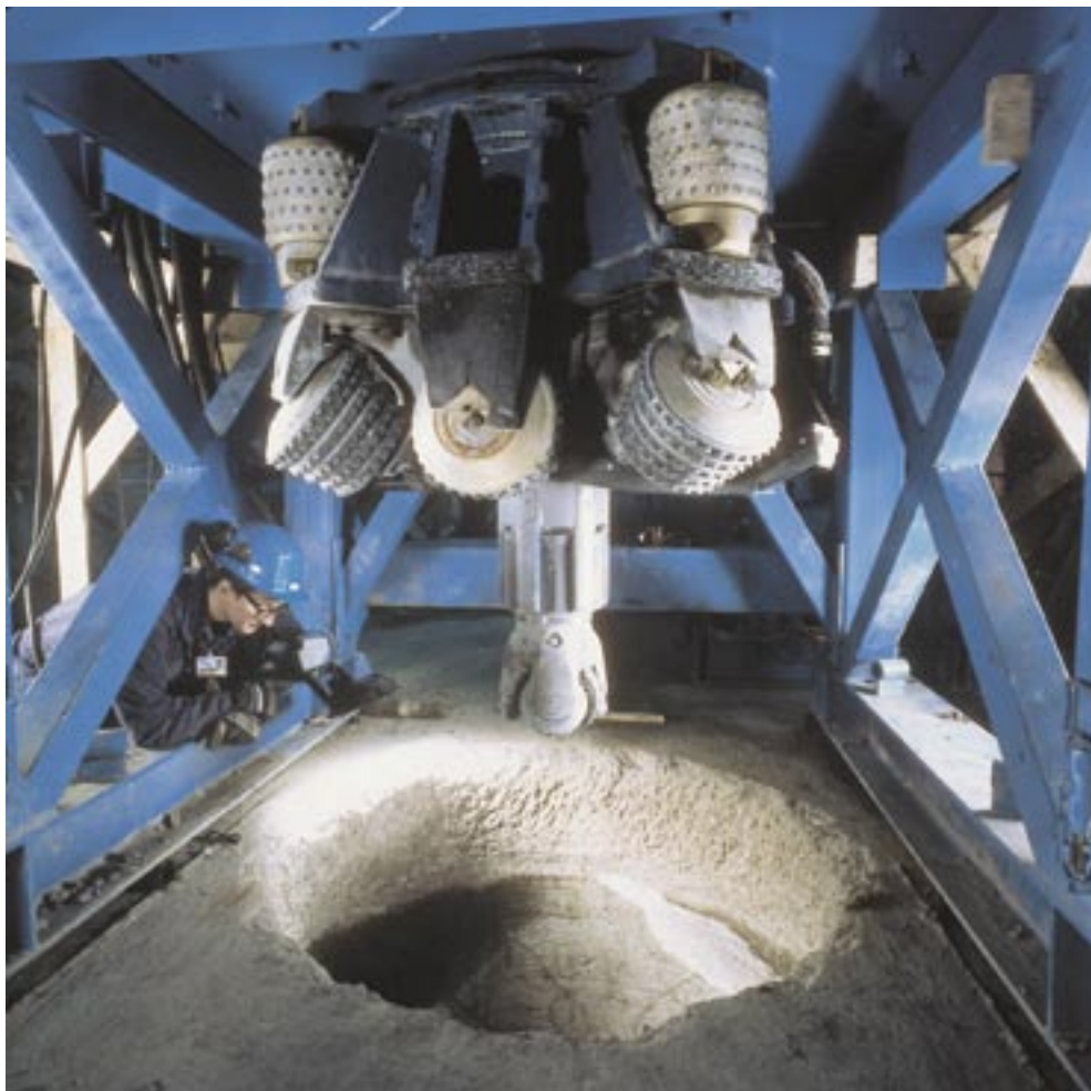
Figure 4-25. Photo of the reamer above the excavated hole /Autio and Kirkkomäki, 1996/.
