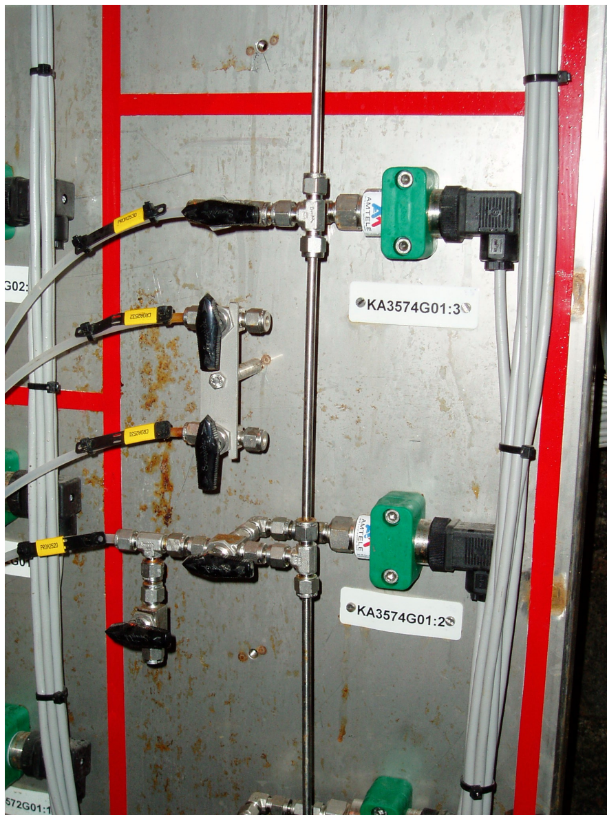
Figure 4-2 Pressure transducers connections
