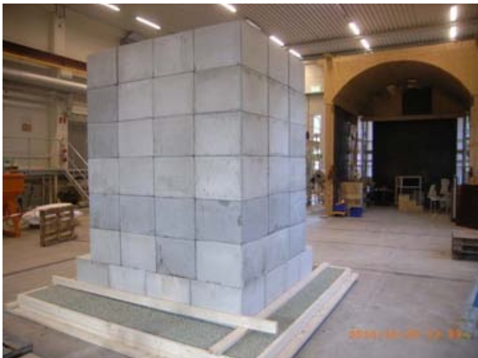
Figure 6-1. Stacking of blocks after a given pattern on a not compressed bed of pellet materials.
