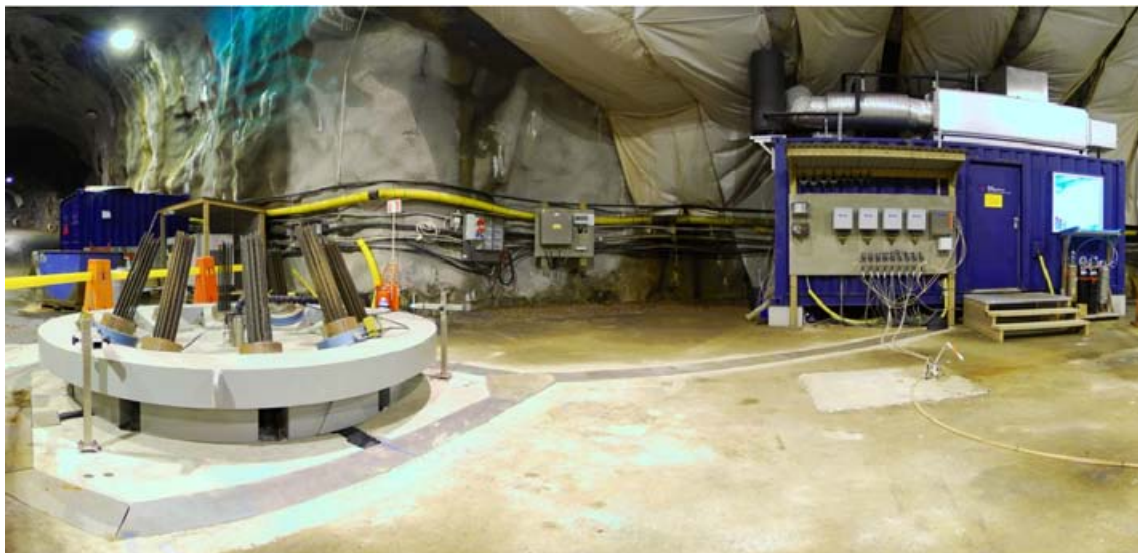
Figure 4-16. The Large scale gas injection test at the –420 m level in Äspö HRL.
