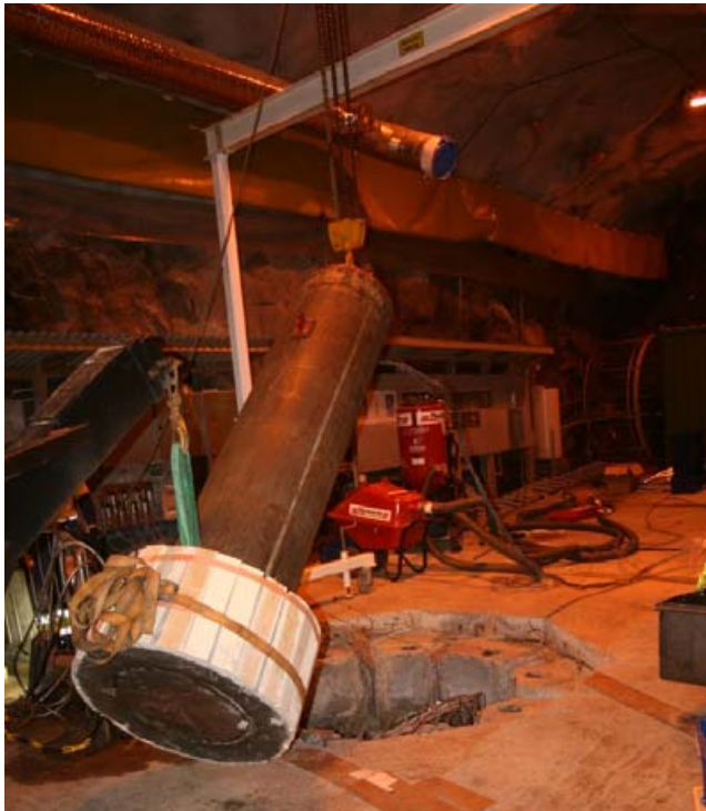
Figure 4-11. Lifting of Heater 1 with attached bentonite material from Ring 1. This material constitutes an undisturbed bentonite-iron interface sample.
