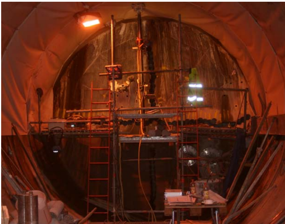
Figure 4-5. The outer plug in the Prototype Repository in December 2010 with the core drilled holes.
