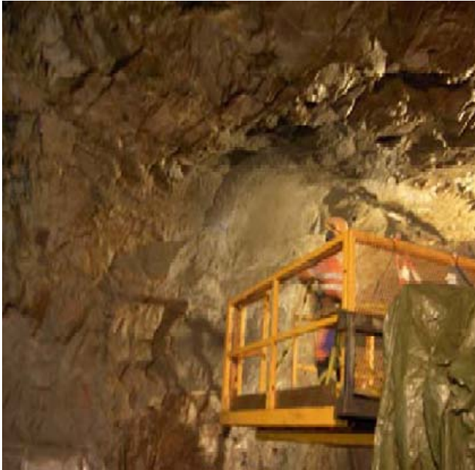
Figure 4-24. Filed test with low-pH shotcrete at Äspö HRL.
