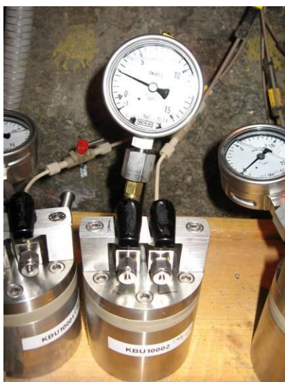
Figure 4. Pressure vessels used for extracting pore water and gas from the Prototype repository.
