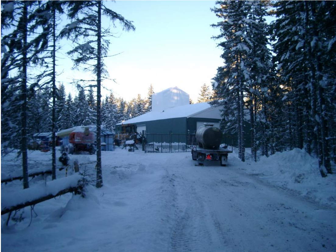
Figure 1-5. Drilling site DS2 at Forsmark. To protect the water system and other sensitive equipment from freezing, a tent with electrical heaters was used to keep the temperature above zero. Another advantage with the tent was improvement of the working environment.
