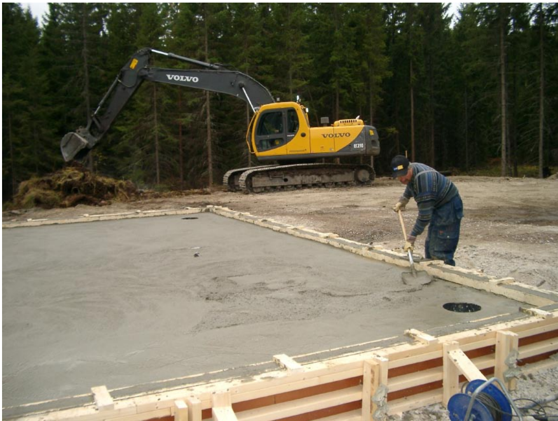
Figure 1-4. The mapped outcrop was filled with gravel and a 7 x 5 m cement slab was cast around the planned collaring point of the borehole.
