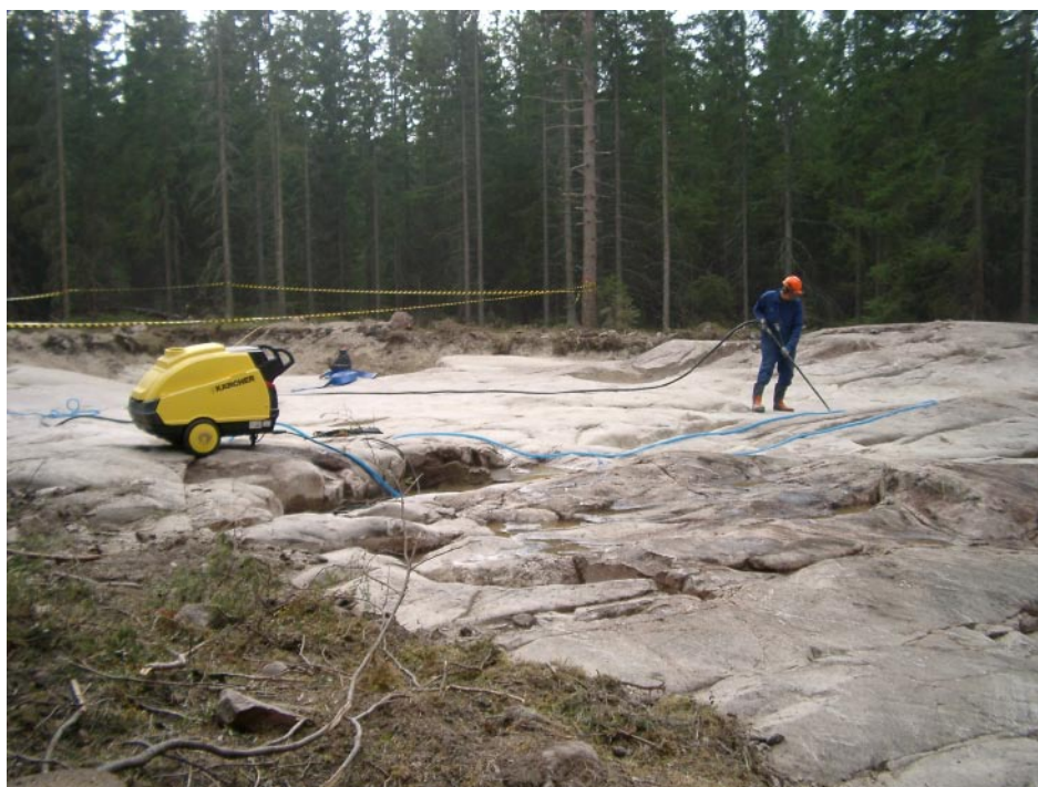
Figure 1-3. Overburden was removed and the bedrock cleaned at drilling site DS2.
