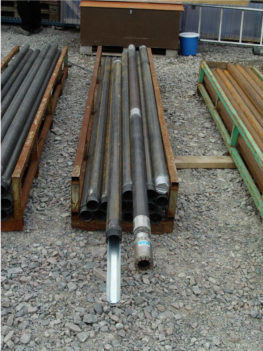
Figure 4-2. For core drilling of KFM02A a 3 m triple tube WL-76 system was used. With the technique applied, a high core quality was obtained. The system provides a borehole diameter of \text{Ø } 77.3 , and the core diameter is 50.8 mm. To the right, a complete core barrel with drill bit and reamer. To the left, the inner tube with one half of the split tube.
