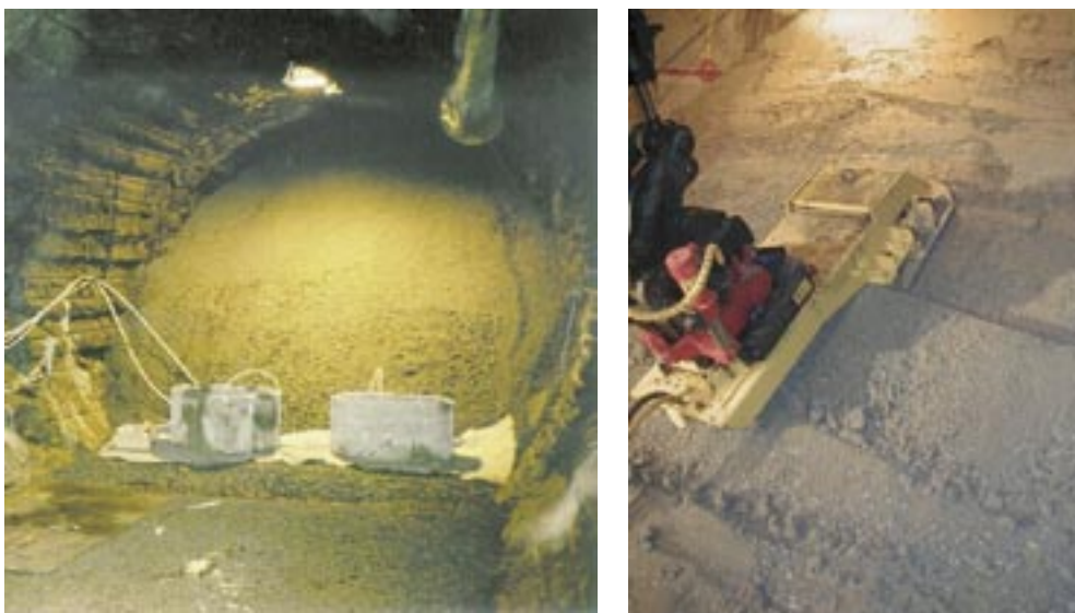
Figure 7-1. Backfill of crushed rock and bentonite. Left photograph shows Backfill and Plug test in Äspö Hard Rock Laboratory. Right photograph shows in situ compaction in Prototype repository in Äspö HRL.
